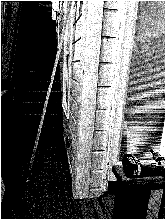
Photo C: Replaced siding, prior to painting
