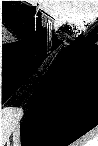
Figure 13: West roof gutter. Note water ponding locations
