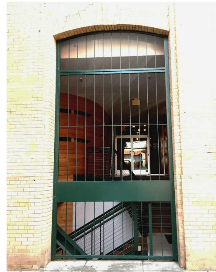
TRANSPARENCY/GATES WITHIN DISTRICT 55 Union St.
