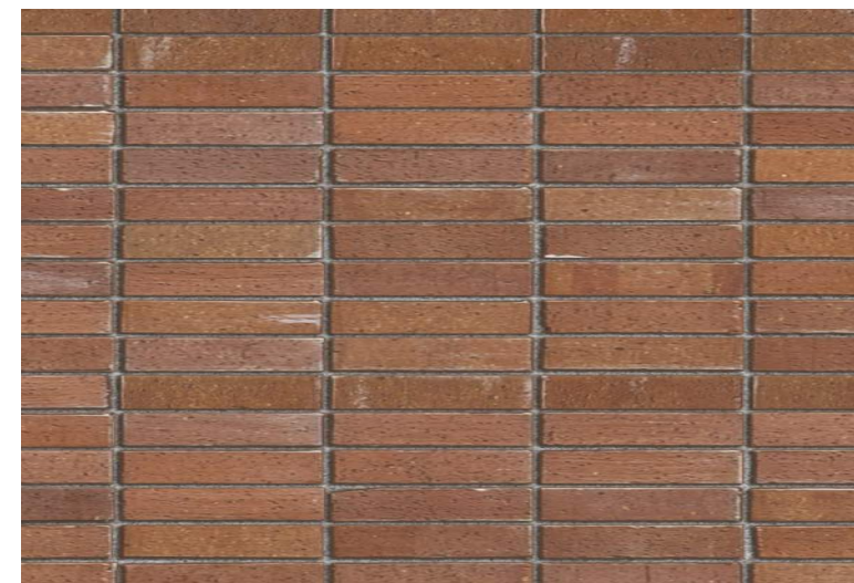
STACK BOND BRICK WALL
