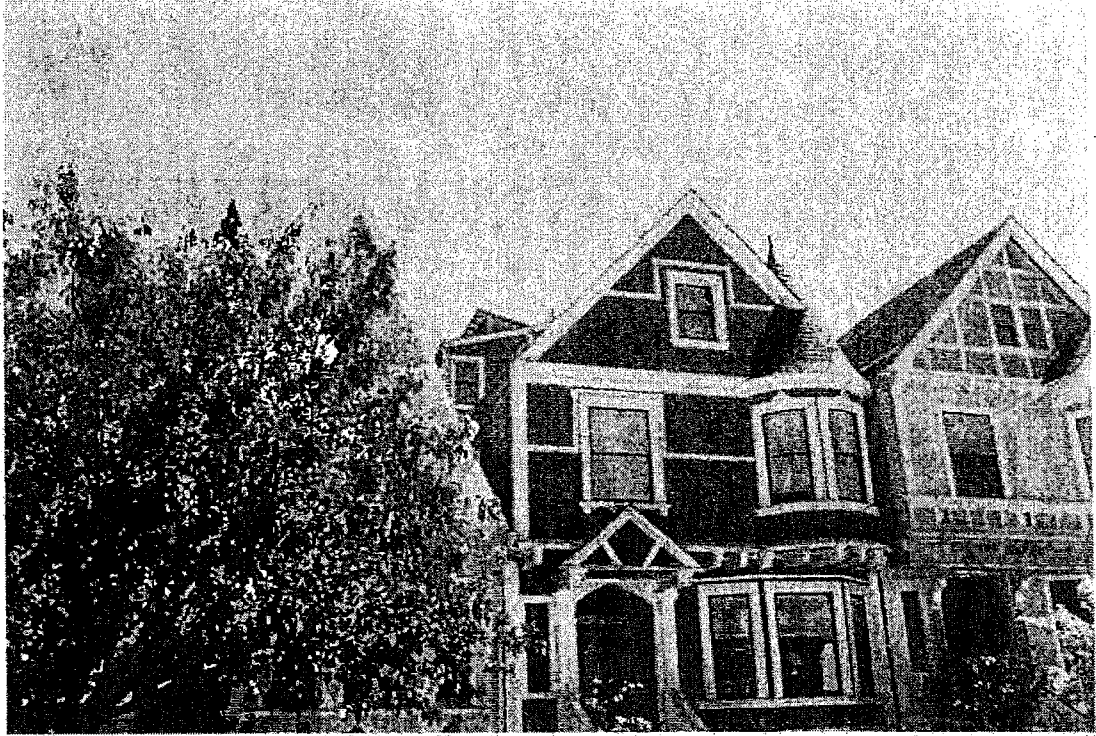
64 Pierce Street roof and facade
