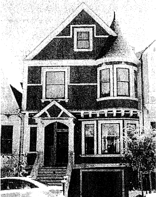
64 Pierce Street facade
