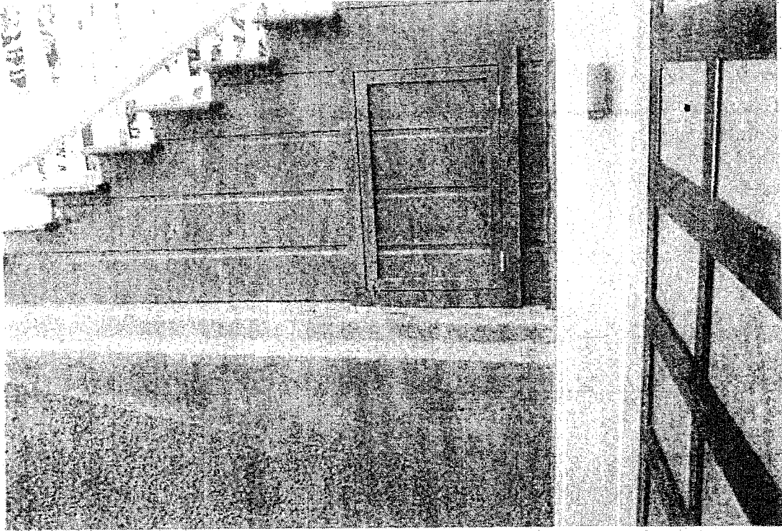
Siding below entry stair, stucco wall finish and permeable concrete driveway
