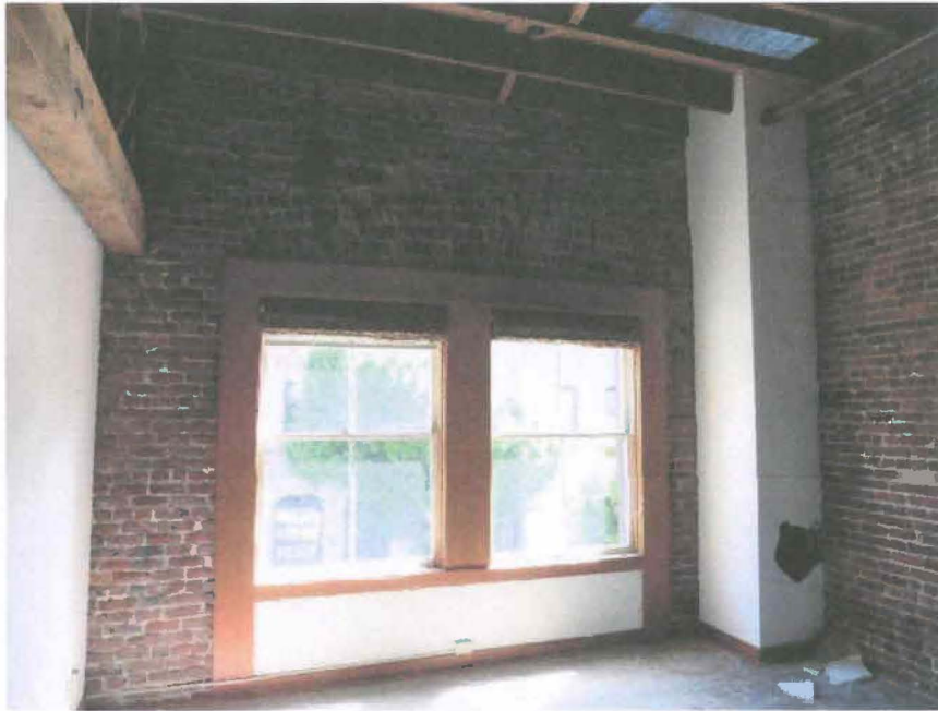
Interior of Montgomery Street 2 nd Floor windows
