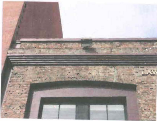
Montgomery Street Cornice Detail
