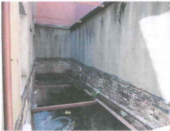
Rear Courtyard with bracing
