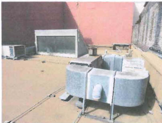
Roof, looking southwest
