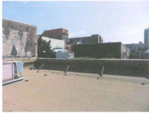
Roof with parapet braces
