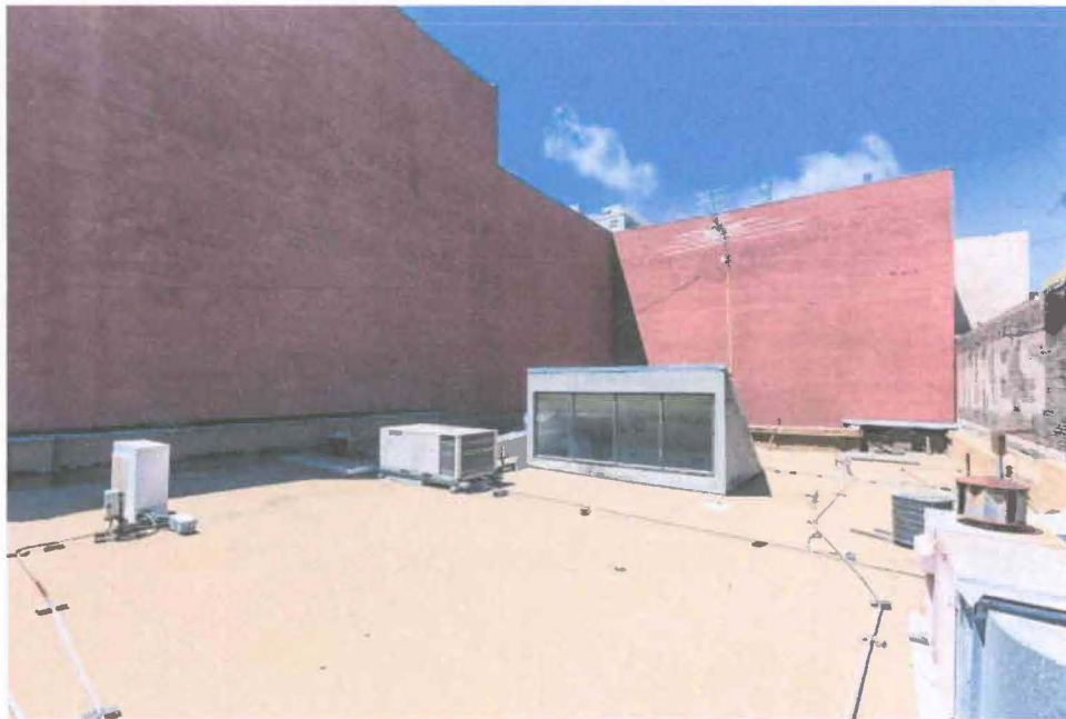
Roof Overall, looking west
