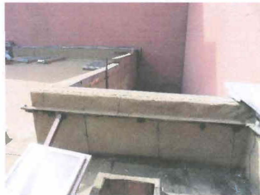
Roof and rear courtyard parapet
