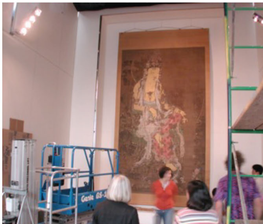
Kagami Jinjya Exhibition Installation - A new interior wall and display case was built over the glass curtain wall of the North Atrium to display this exhibit.
