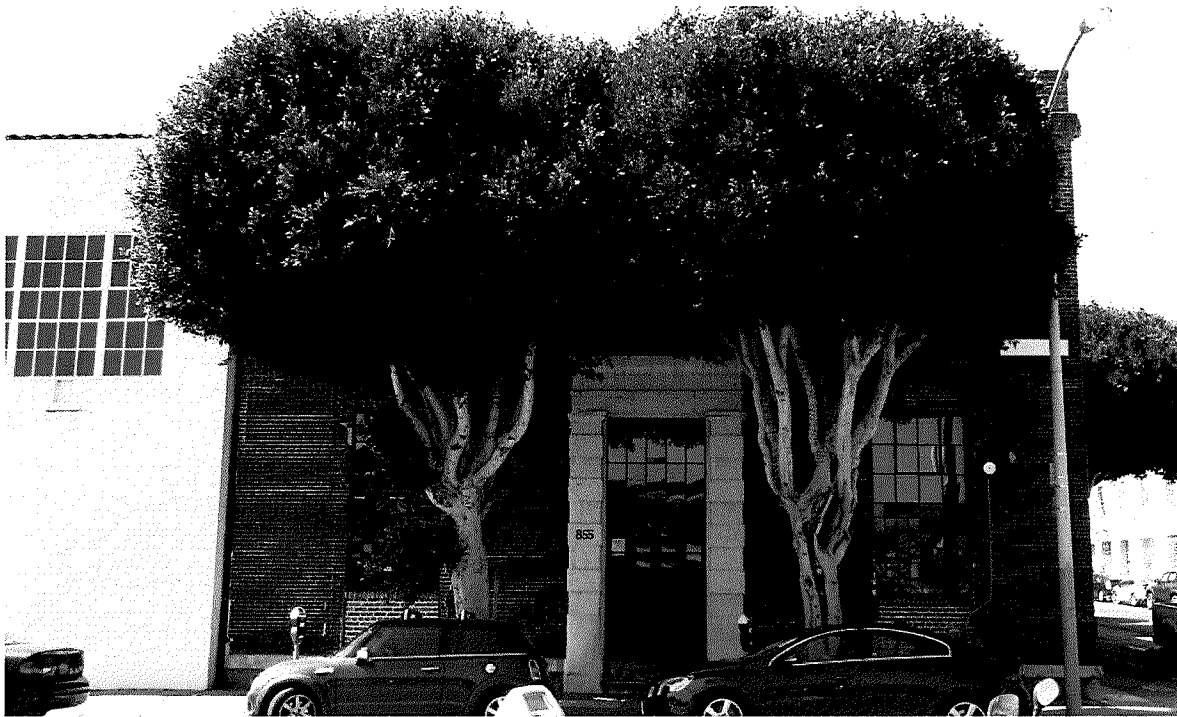
Figure 3 855 Front Street (photography taken on 03/30/2017).
