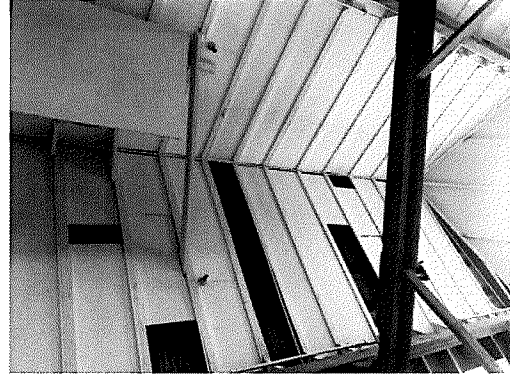
Photo 2: Underside of steep slope roof.
