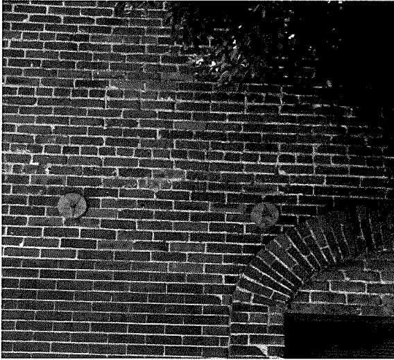
Figure 13 Detail of brick along Front Street (photography taken on 03/30/2017).
