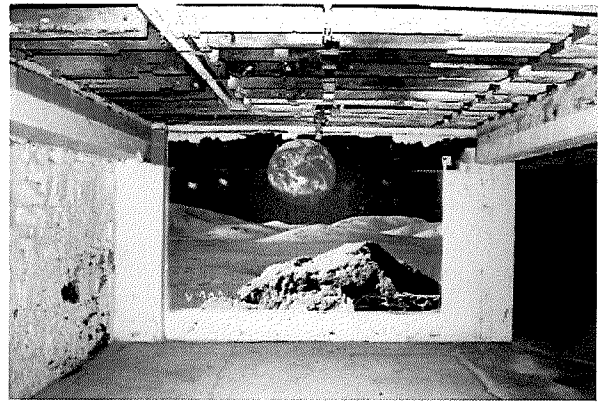
Figure 116 Extant mural in the basement level, not historic (photograph taken on 04/04/2017)
