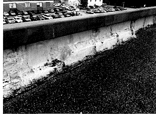
Photo 18: Roof sheet extends up brick parapet.
