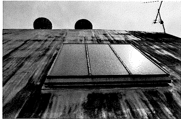
Figure 49 Detail photograph of skylights on steep-pitched roof (photography taken on 04/04/2017).
