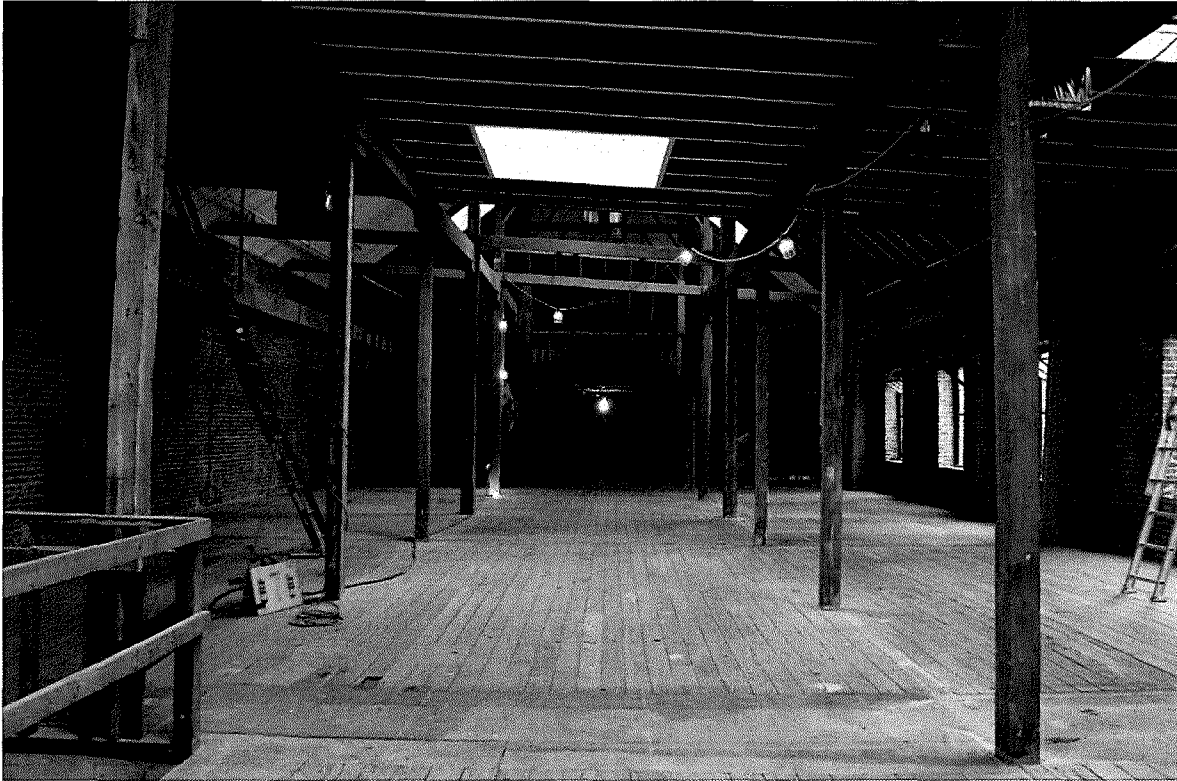
Figure 79 Interior photograph of upper level and attic space (photography taken on 04/04/2017).
