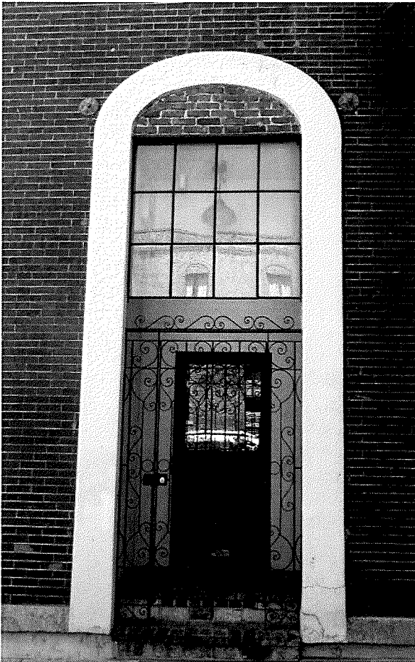
Figure 19 Photograph of easternmost entrance on Vallejo Street (photography taken on 03/30/2017).
