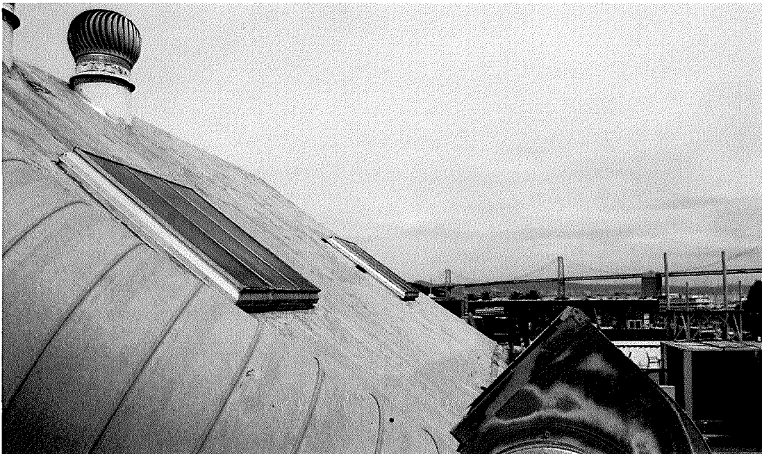
Figure 5 Photograph of eastern side of hipped roof (photograph taken on 04/05/2017).
