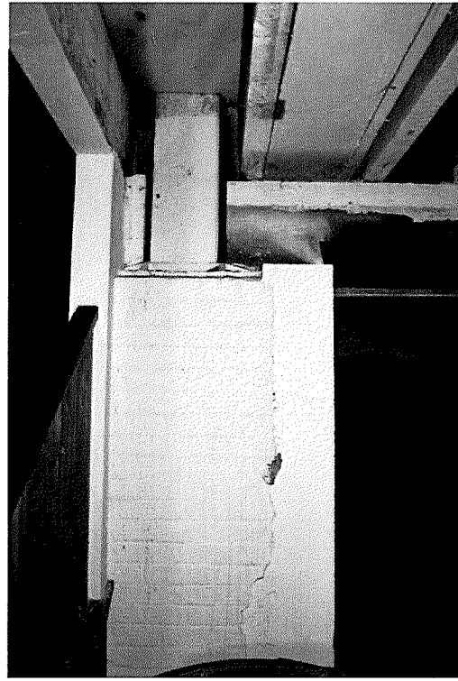
Figure 70 Detail of structural brick pier. Note parging cement (photography taken on 04/04/2017).
