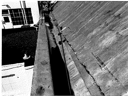
Photo 10: Perimeter drainage trough at base of steep slope.
