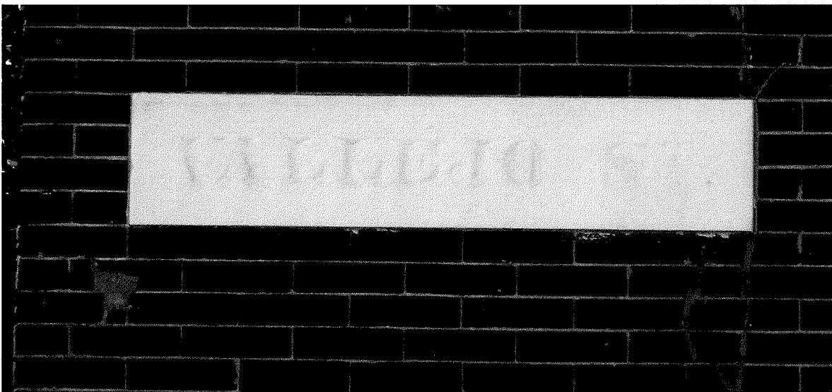
Figure 36 Detail of street signage on the Front Street elevation (photography taken on 03/31/2017).
