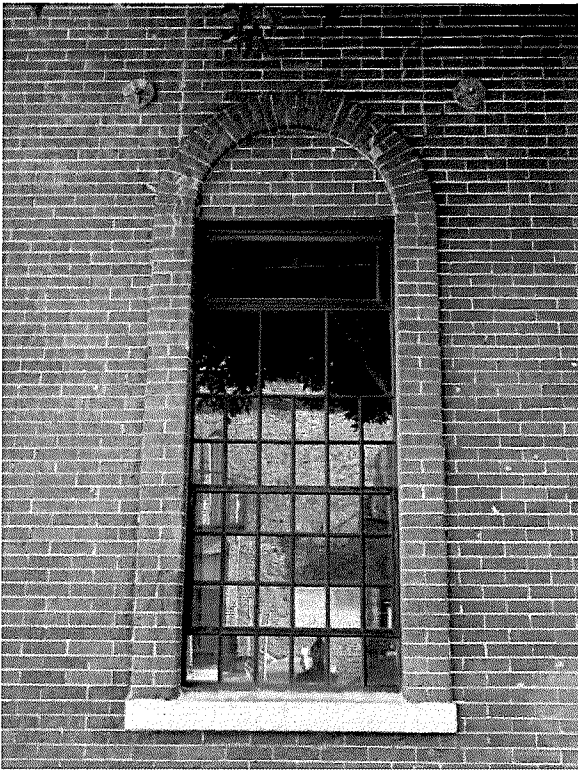
Figure 24 Historic ground level window type. Note transom glass, metal frame, brick surround, and granite sill (photography taken on 03/31/2017).
