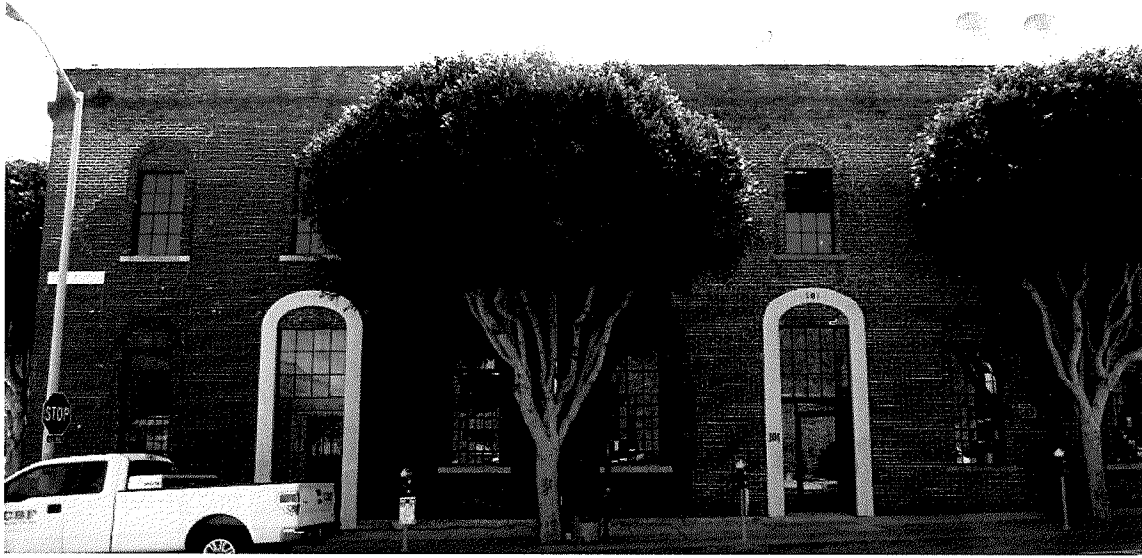
Figure 95 Photography of Vallejo Street elevation. Note characteristic differences between brick of different eras (photograph taken on 03/30/2017).
