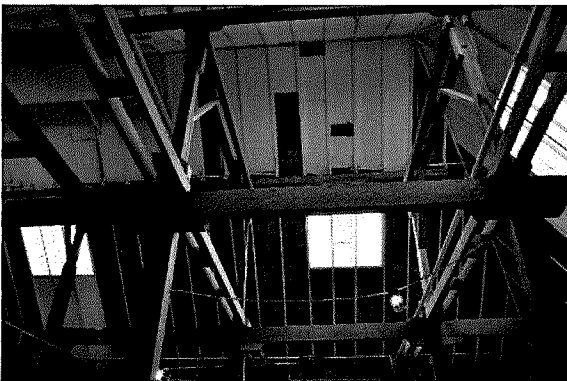
Figure 122 Detail view of structural timber construction at the upper level (photograph taken on 04/04/2017).
