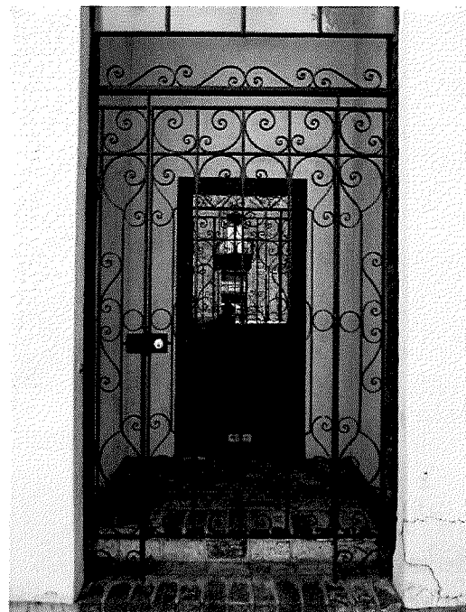
Figure 97 Detail photograph of easternmost entrance along Vallejo Street. Note stucco over brick threshold, metal security gate, and modern aluminum frame door (photograph taken on 03/30/2017).
