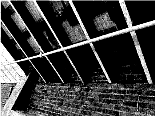
Photo 3: Underside of steep slope roof.
