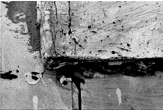
Figure 47 Detail photograph of roof waterproofing construction. Materials include tar, sheet metal, and titanium synthetic underlayment (photography taken on 04/05/2017).
