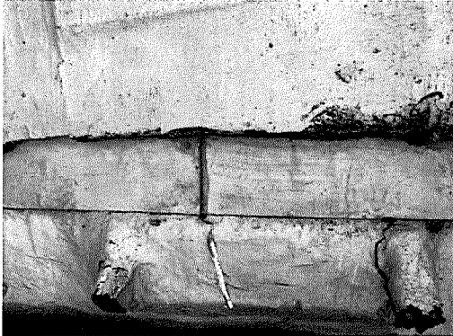
Photo 11: Sheet metal base flashing below the base of the steep slope roofing at the perimeter drainage trough.
