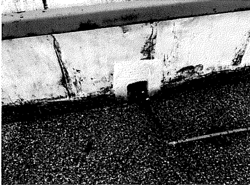
Photo 21: Through wall scupper.
