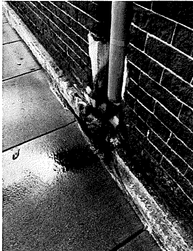
Photo 23: Outlet of downspout at sidewalk.
