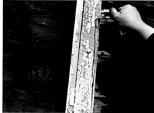
Photo 8: Severe decay in roof framing members.
