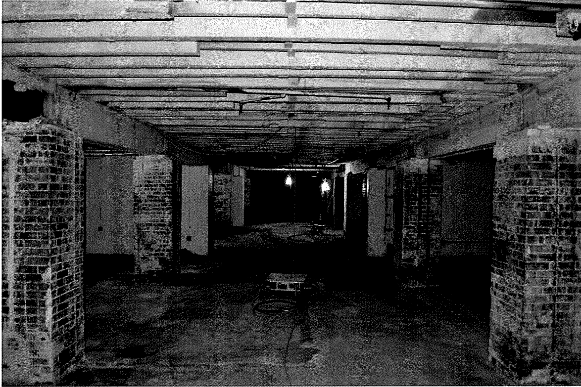
Figure 68 Interior photograph of basement space (photography taken on 04/04/2017).
