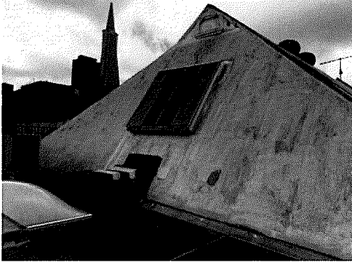
Photo 1: Overview of steep slope roof.
