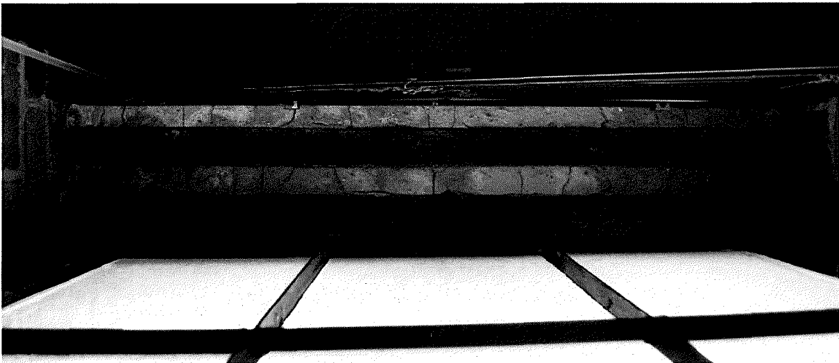
Figure 111 Detail view of lintel construction at window openings. Note cracking of parging coat typical (photograph taken on 04/05/2017).
