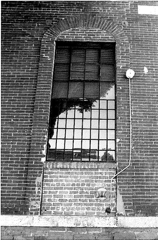
Figure 10 Detail of window opening along Front Street (photography taken on 03/30/2017).
