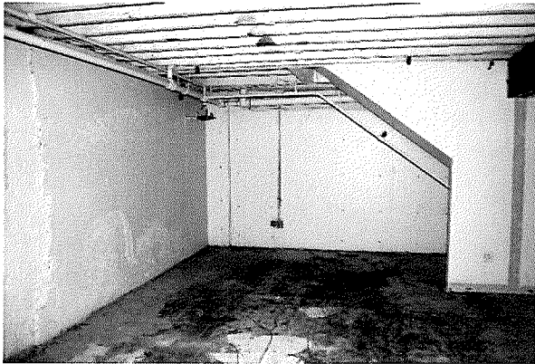
Figure 115 Interior photograph at the basement. Note seam between concrete and stone foundations (left). Photograph was taken on 04/04/2017.
