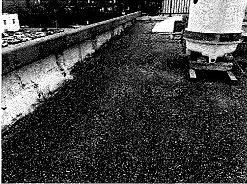
Photo 17: Low slope roof with built-up roof (BUR) and gravel topping.
