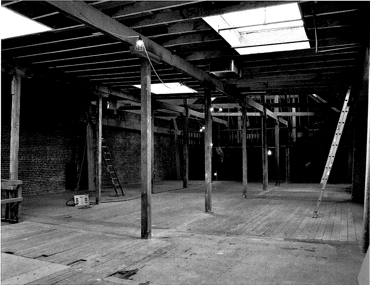
Figure 121 Interior photograph at the upper level, looking east (photograph taken on 04/04/2017).
