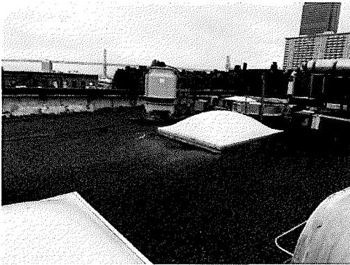
Photo 19: Several pieces of equipment and skylights on low slope roof.
