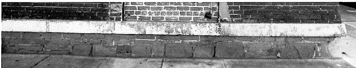
Figure 4 Detail view of foundation stone on Front Street (photography taken on 03/30/2017).
