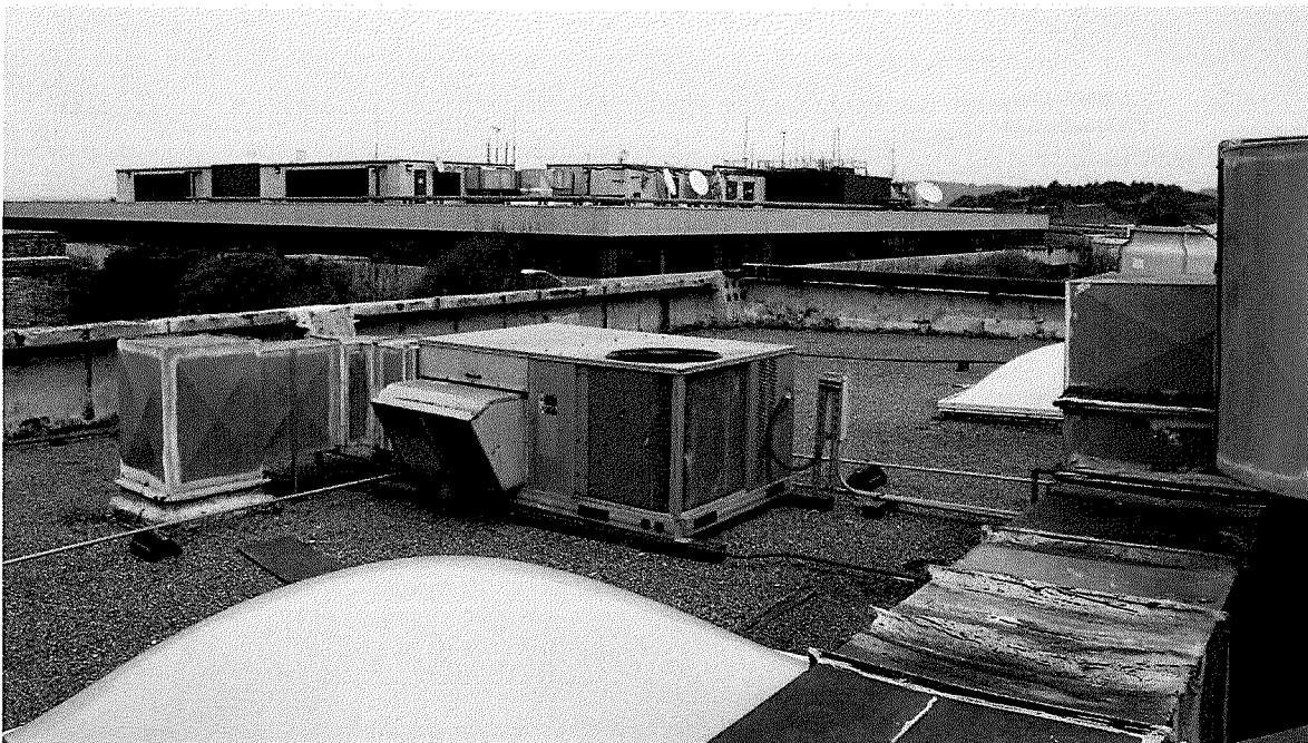
Figure 44 Overall photograph of roof at 101 Vallejo Street (photography taken on 04/05/2017).
