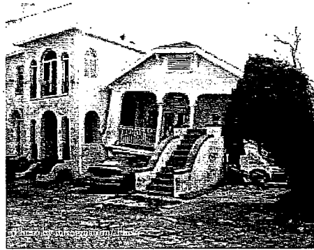
The result of a soft story collapse.
