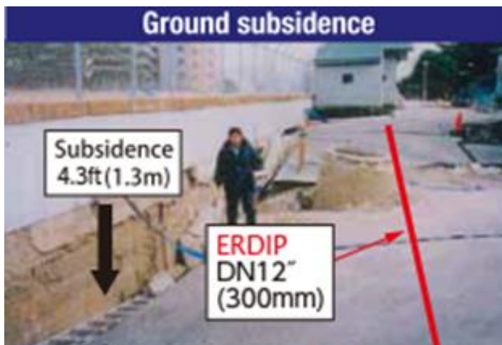
Figure 2 Earthquake Resistant Ductile Iron Pipe (Source: Kubota Pipe)
