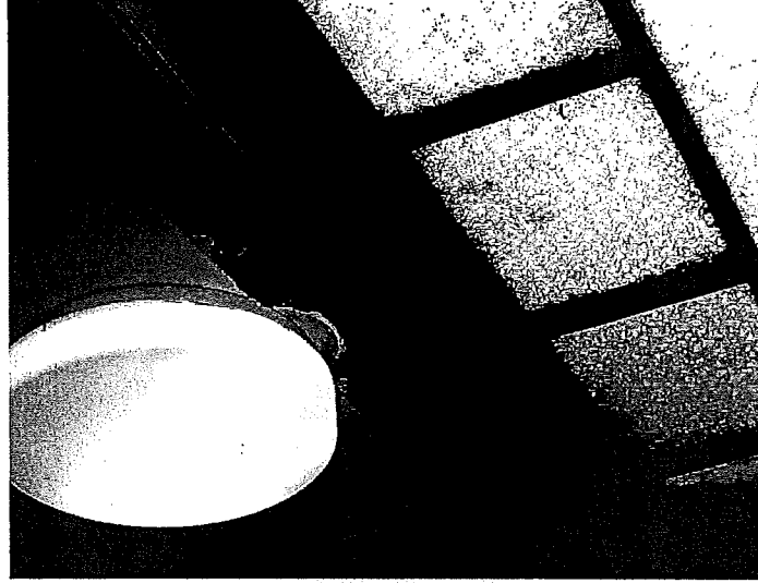
Figure 10: Skylight of textured wire glass has no weatherstripping or putty. Debris has collected on glass. Light fixture cuts into wood frame.
