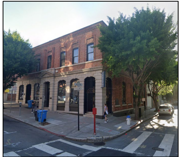
Constructed in 1854, the "Bank of Lucas, Turner & Company" building located at 800 Montgomery Street is San Francisco Landmark #26.
