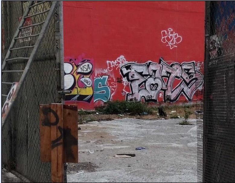
Vacant lot vandalism
