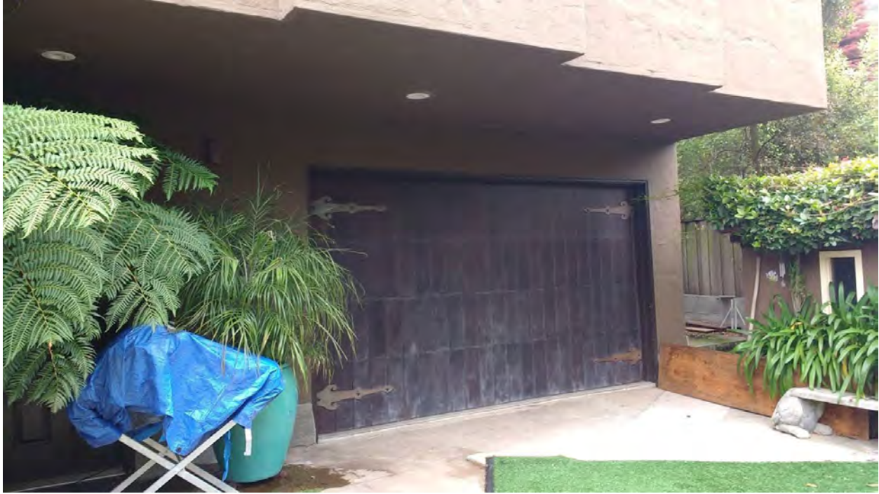
Figure 25. Basement level of northeast façade.
