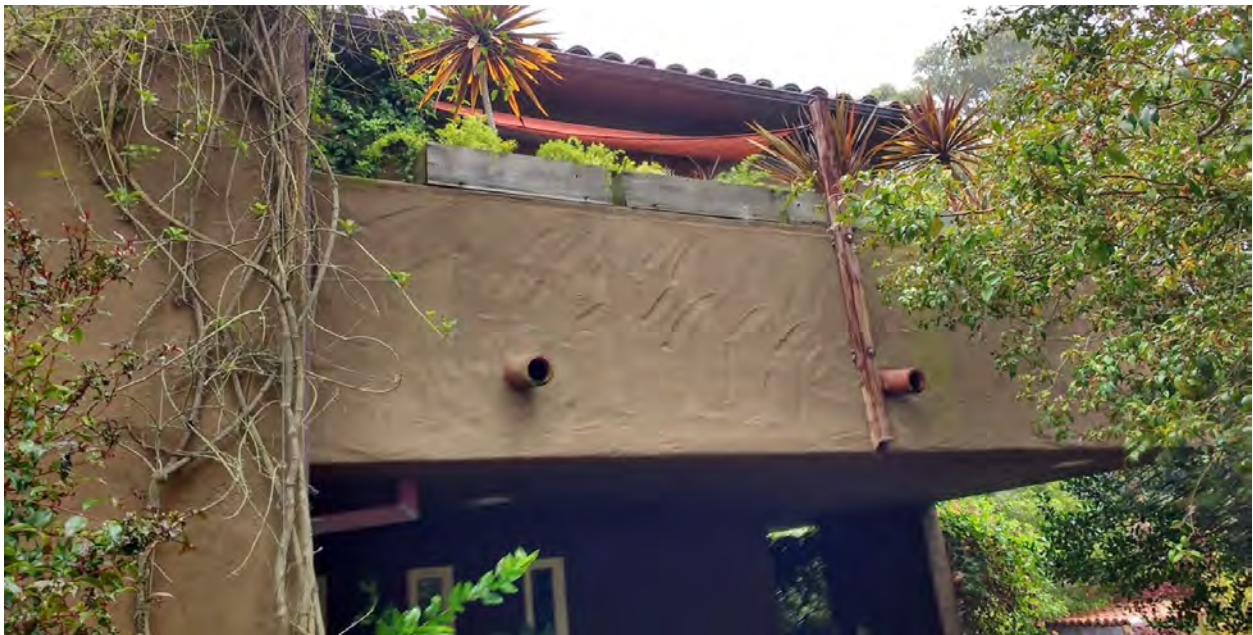
Figure 29. Right side of southeast façade.
