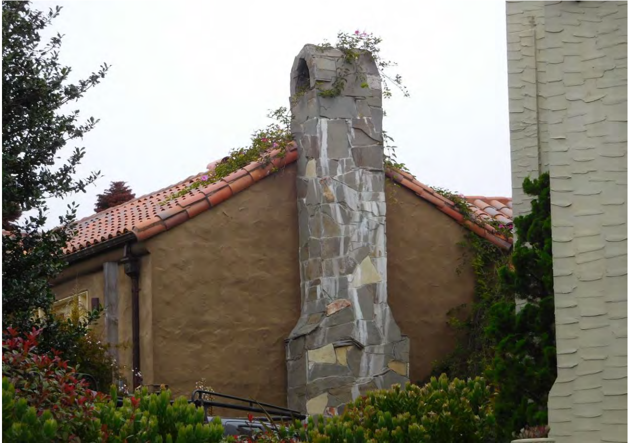
Figure 28. Portion of southeast façade visible from Ventura Avenue.
