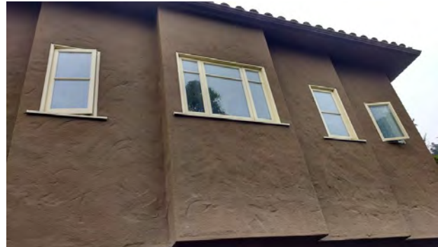
Figure 27. Northeast façade; right side of first floor level.
