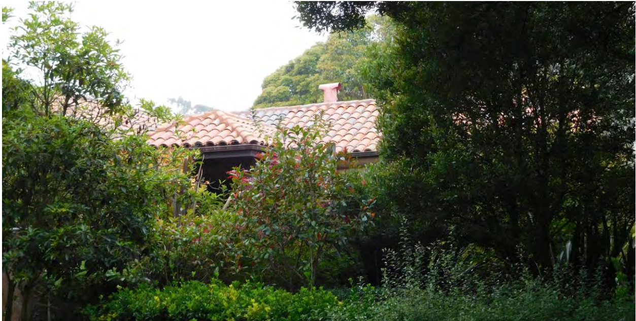
Figure 21. Primary façade of 35 Ventura from street.
