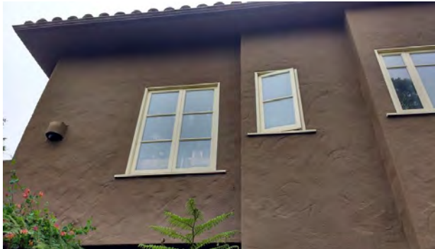
Figure 26. Northeast façade; left side of first floor level.
