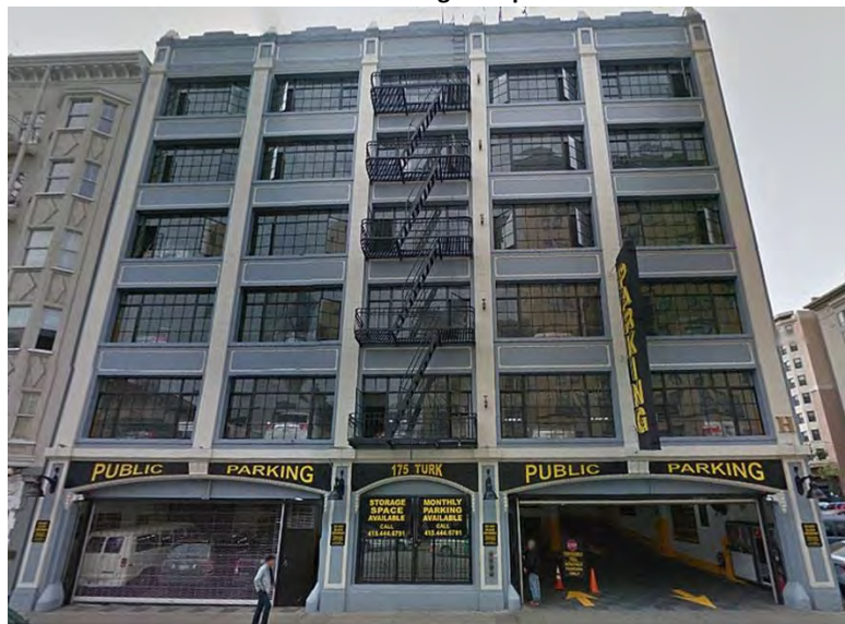
Figure 41. Bell Garage, 175 Turk Street. Source: Google Maps
