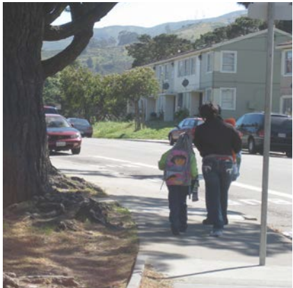
Sidewalk at Santos Street near Sunnydale. Tree roots have damaged some sidewalks in the neighborhood.
