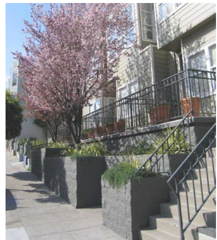
Townhouses above street due to grade change
