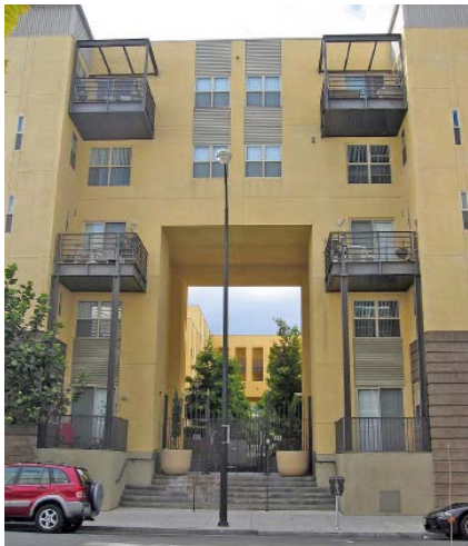
Shared portal entry
