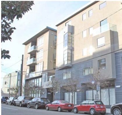
Examples of significant breaks
