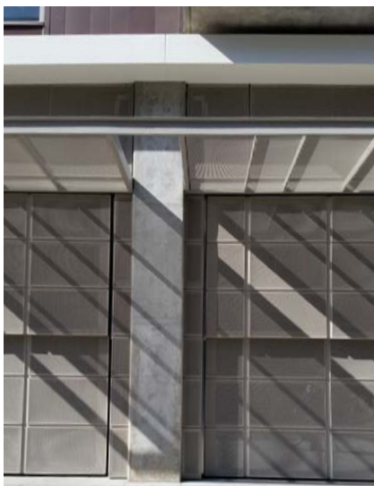
Garage entry and screening designed to integrate with architecture.
