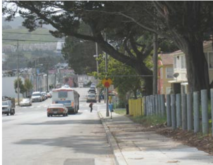
C View looking south along Hahn Street.
