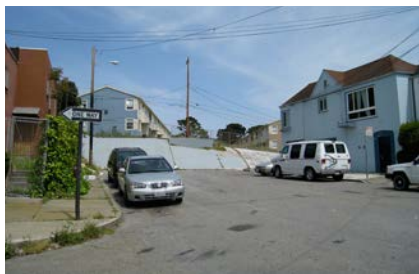
Discontinuous street and barrier at Carrizal
