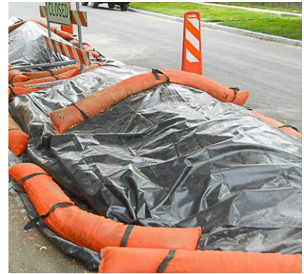
Construction pollution prevention
