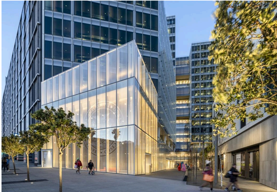
Figure 8: Permit Center at 49 South Van Ness
