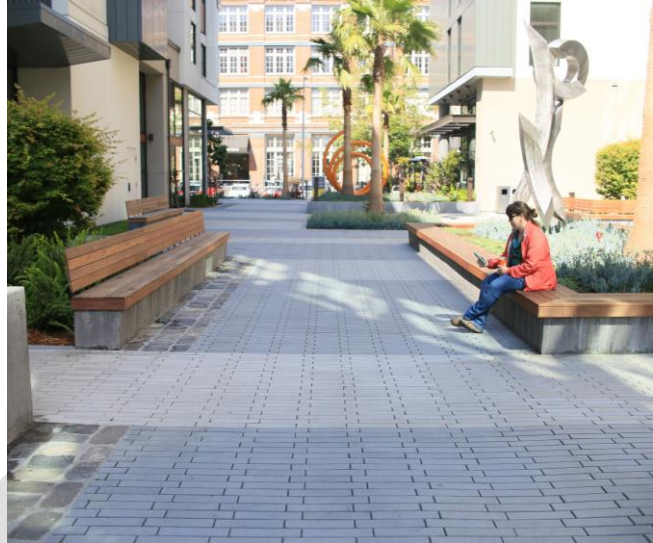
Pervious concrete in parking lot (Presidio, San Francisco)
