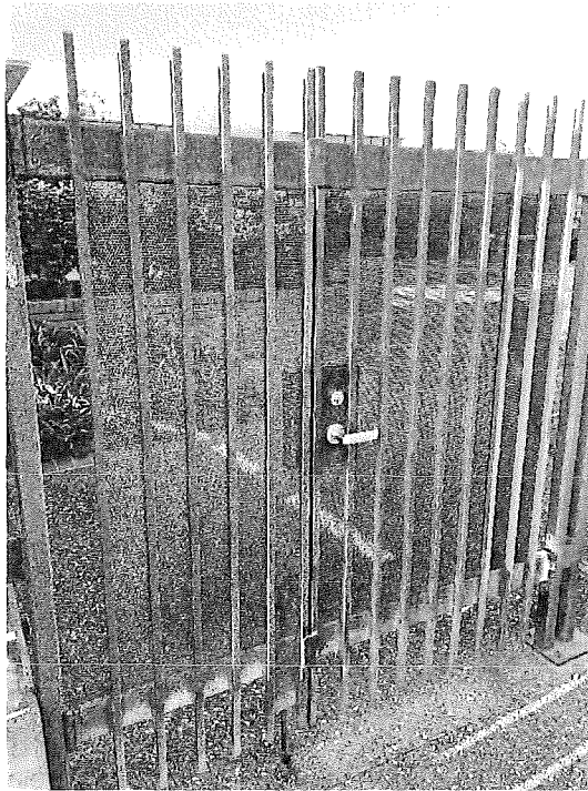
Photo 9: Access from Euclid and Masonic Avenues is restricted by a secured gate which is kept locked and requires a key to open. The gate is the access to the Upper Terrace.
