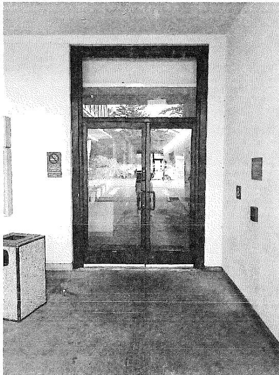
Photo 4: Door from northeast side of the parking lot that leads through the building interior and opens through another secure door into an exterior southeast facing patio area.
