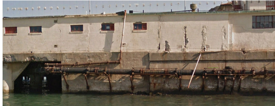
Fort Mason Pier 1
