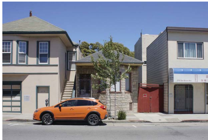
3 SUBJECT PROPERTY FRONT FACADE
