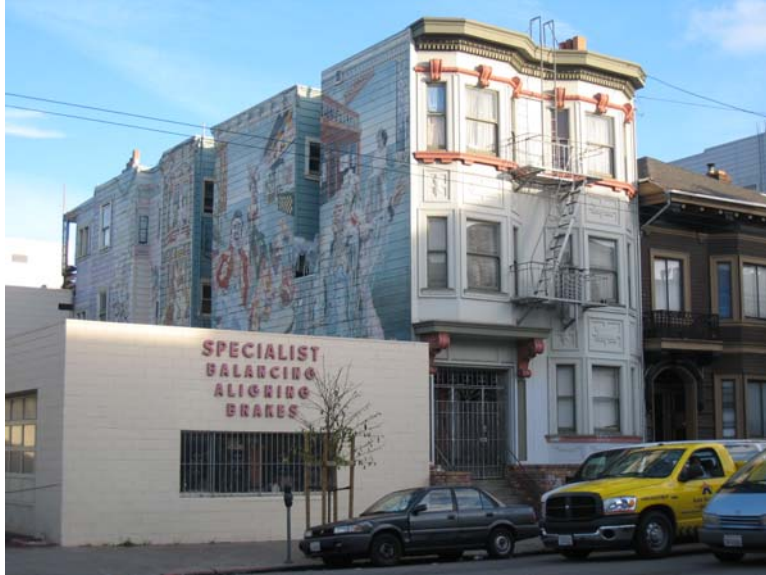
View looking southeast at the north façade. Source: San Francisco Planning Department
