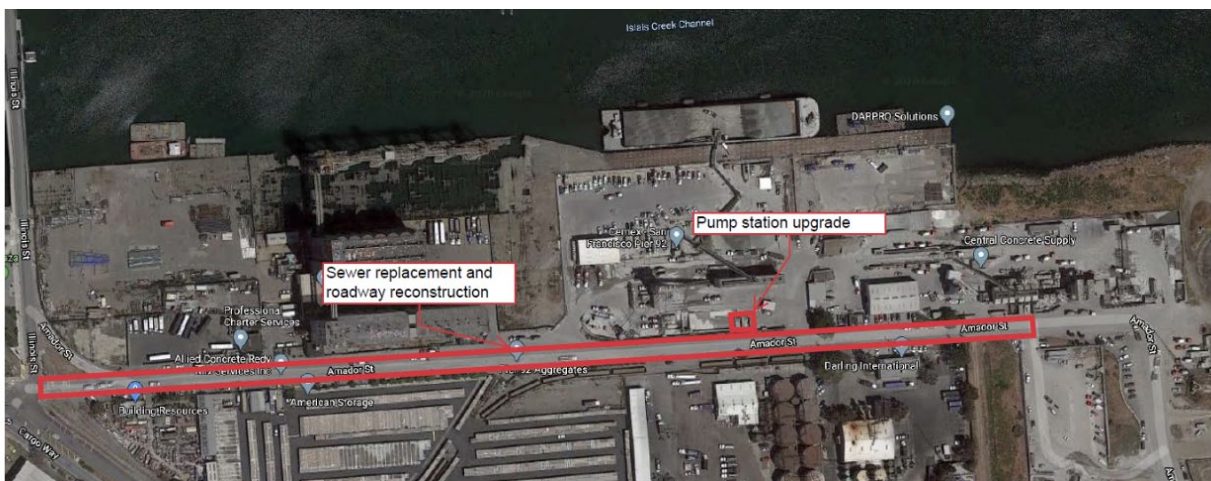
Figure 2. Aerial Overview of Project
