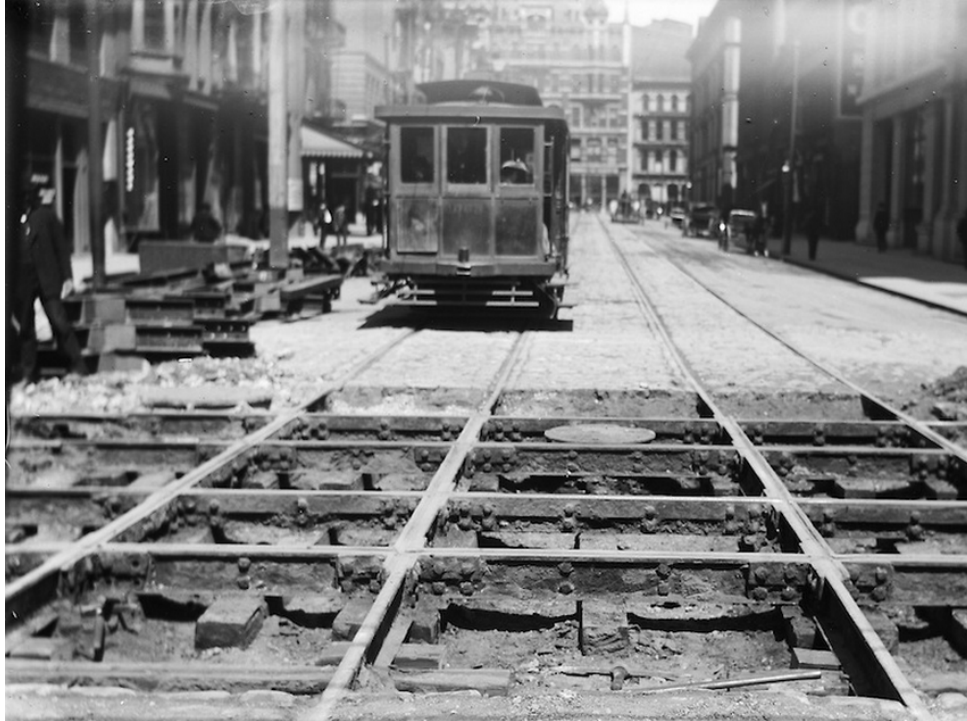
View toward Market Street as a streetcar approaches track construction at Second and Mission, circa July 1904. A small portion of the Burdette Building is visible at the extreme upper left. (SFMTA Photo Archive)
