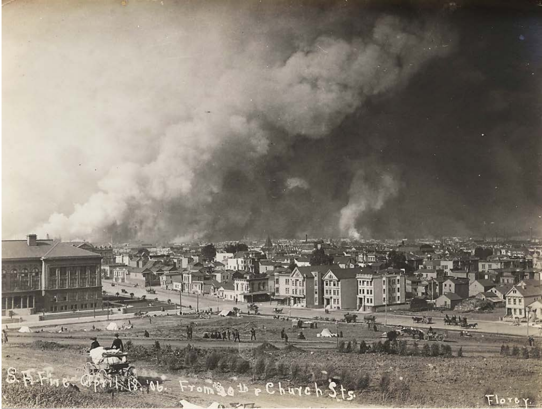
View northeast from Dolores Park of fires in the South of Market and Hayes Valley approaching the Mission District. (Bancroft Library)
