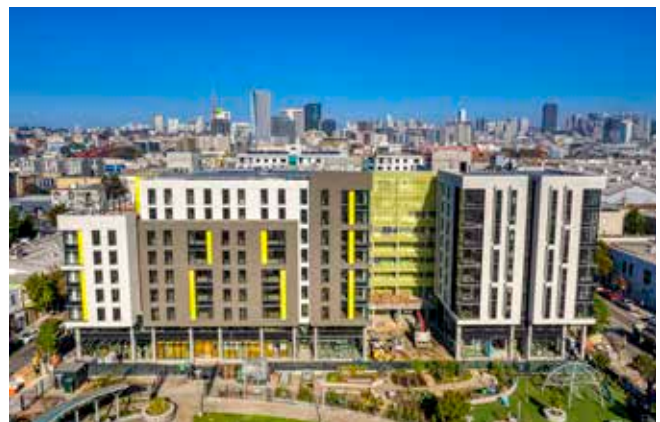
Casa Adelante (2060 Folsom): all-electric affordable housing with 127 affordable apartments, and 29 units for formerly homeless transitional-age youth. Developed by MEDA and Chinatown CDC. Photo credit: James E. Roberts-Obayashi Corp. (general contractor)
