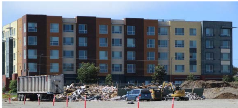
Pictured above is a recent example of illegal dumping/disposal near the Alice Griffith Apartments in the Bayview-Hunters Point neighborhood.
