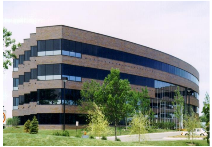
Kensington Office Building
