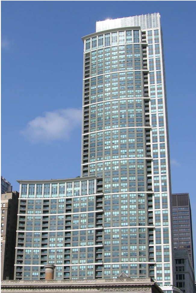
Heritage at Millennium Park
