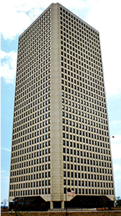
Breakers at Edgewater
