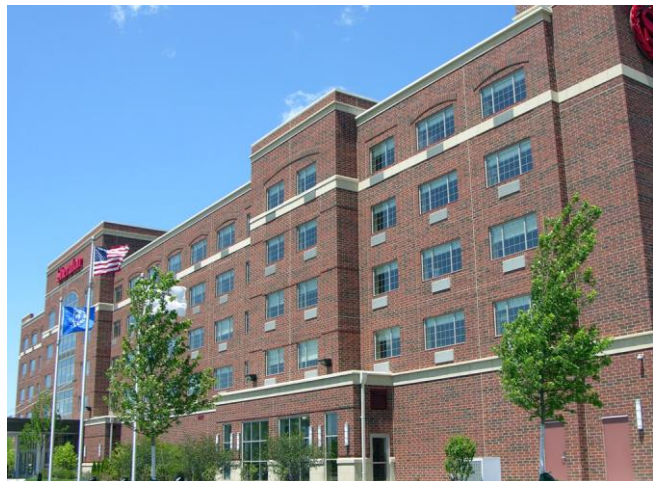
Sheraton Chicago Northbrook Hotel
