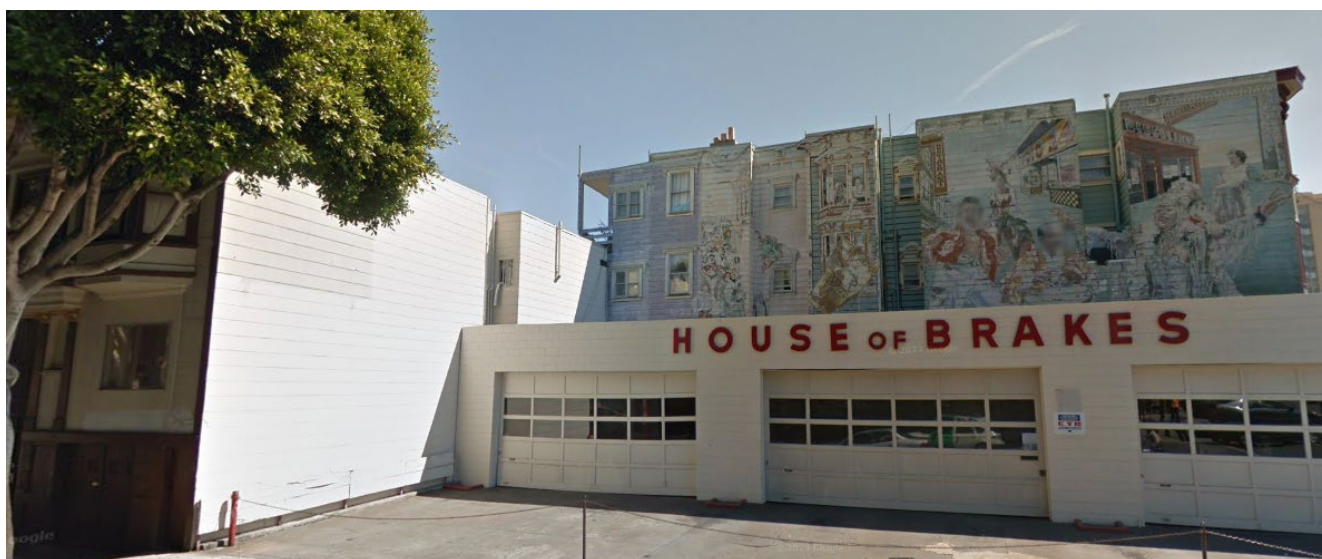
Google Streetview, looking south from 24 th Street, August 2014.
