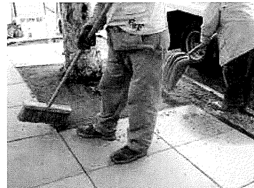
Rubber sidewalk installation
