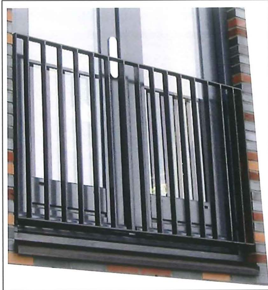
ORNAMENTAL IRON RAILINGS
