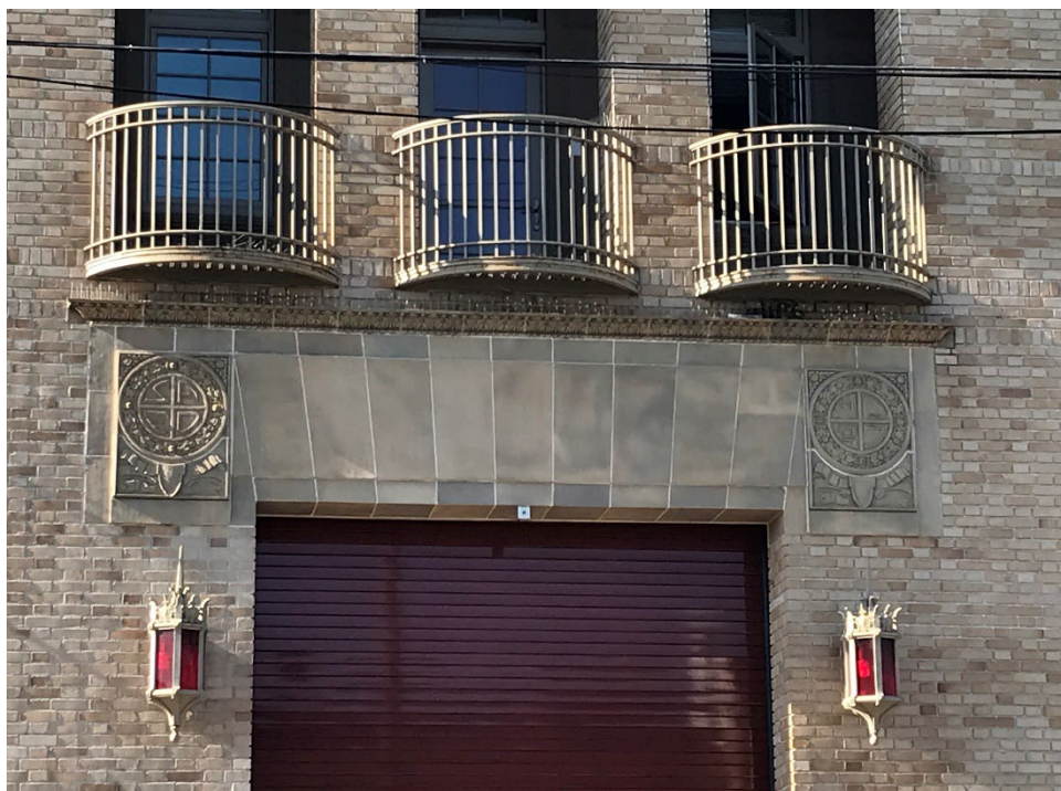
San Francisco Fire Station No. 44, Girard Street façade details, view west, 2023. Source: SF Planning Department
