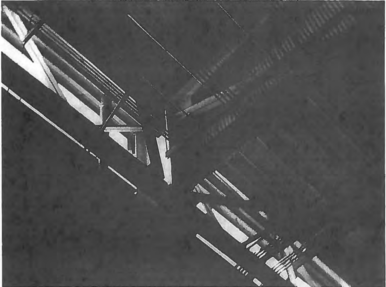
Photo 6. View of the steel column and steel truss connection
