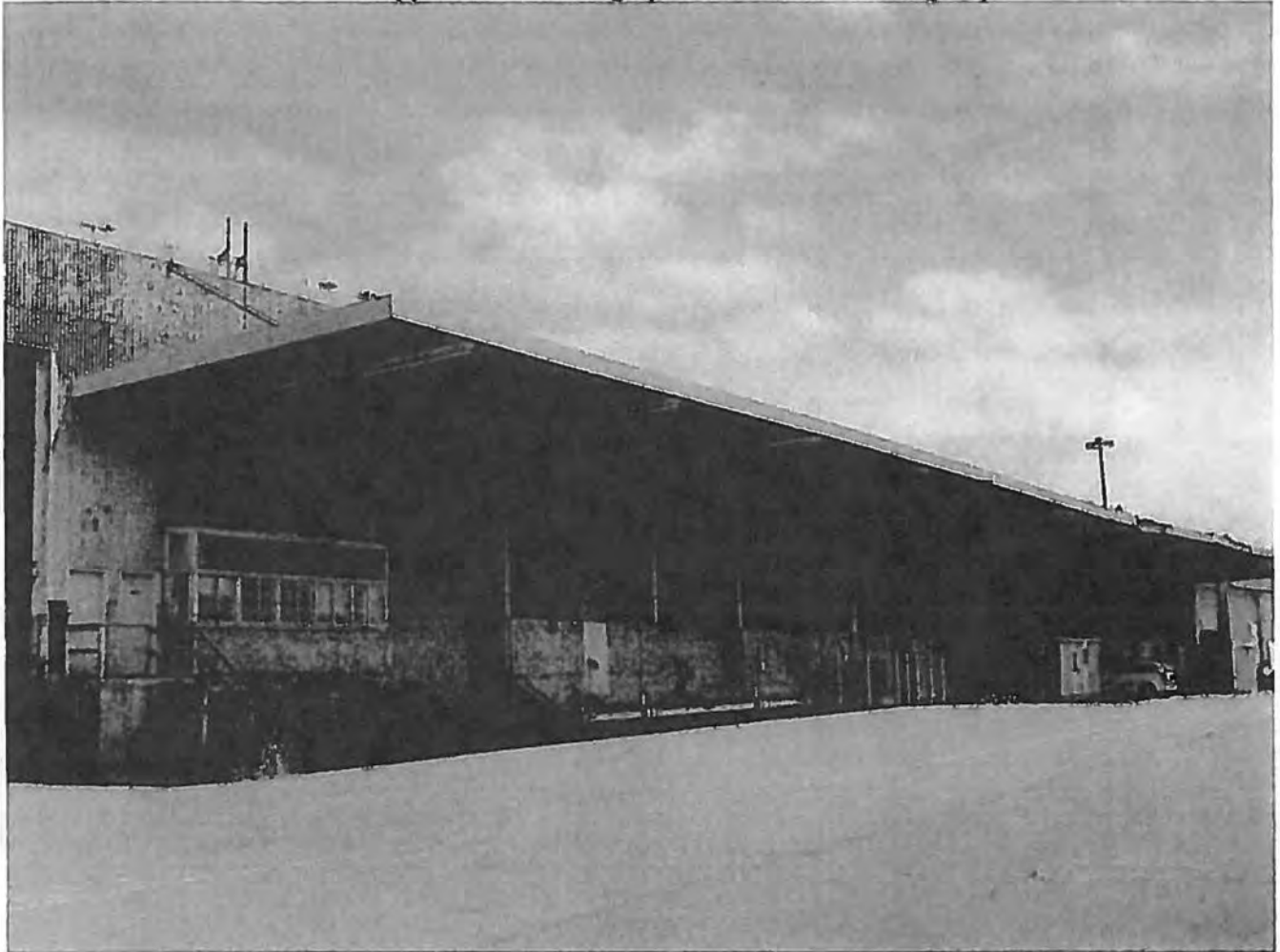
Photo 11. View of the south canopy near the southeast corner
