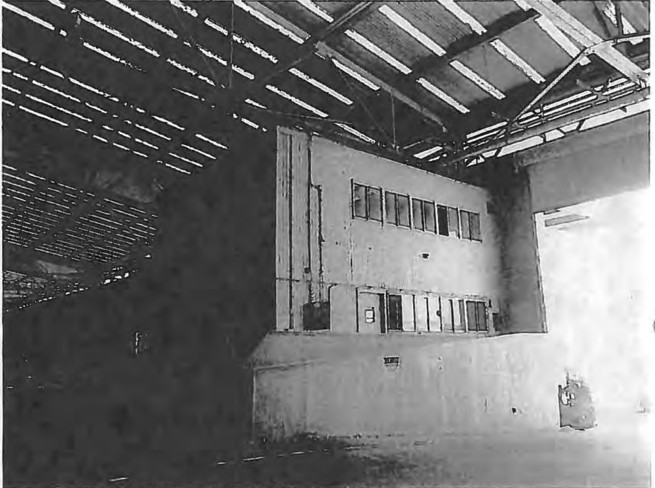
Photo 17. View of the wood-frame structure inside the shed
