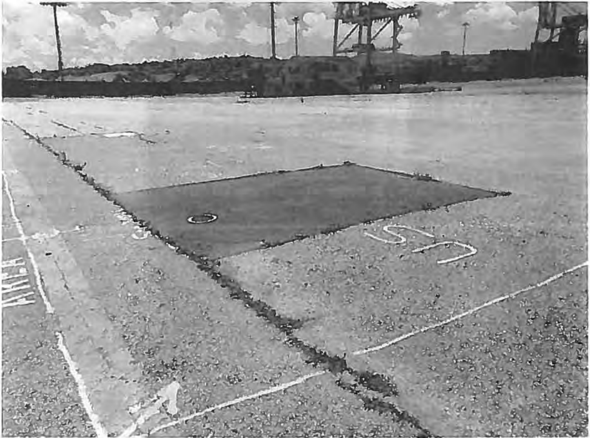
P80 C Face (north) recently repaired underground valve feeding ships water service (Note piping and valve under deck and on face are missing). (Image #20)
