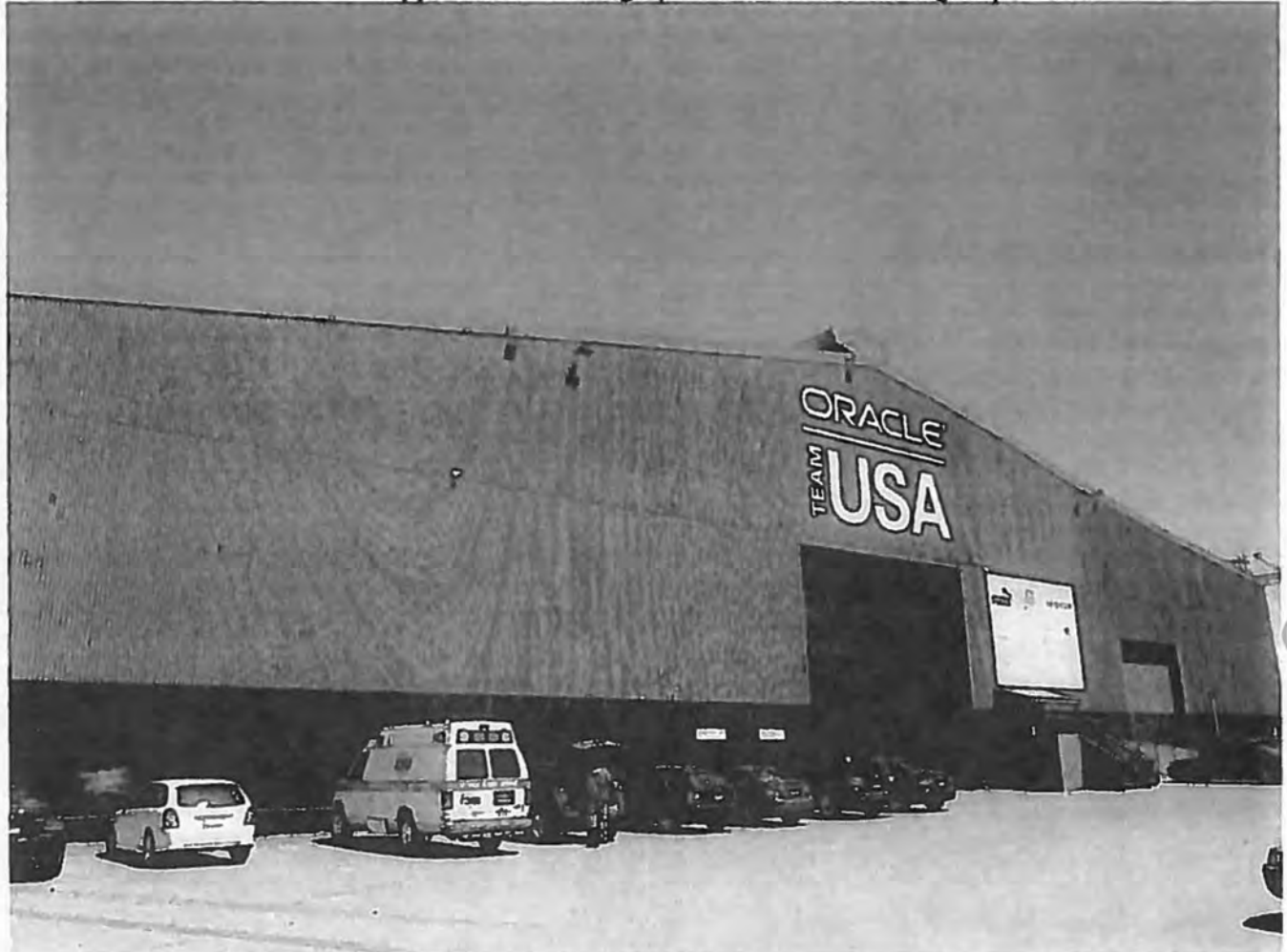
Photo 1. View of the west elevation
