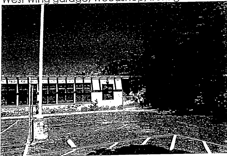
West wing woodshop & gate
