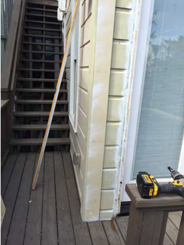
Photo C: Replaced siding, prior to painting
