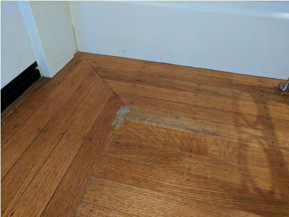
Photo A: Bedroom floor warping (sealed with wax)
