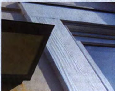
Figure 19: Raised grain at trim
