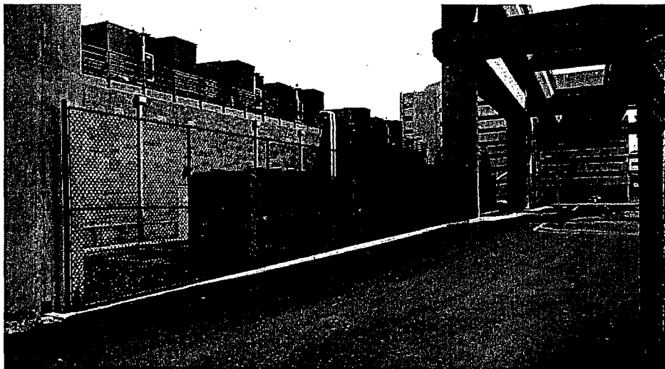
Photo 3C: Airport Data Center (Looking East)
