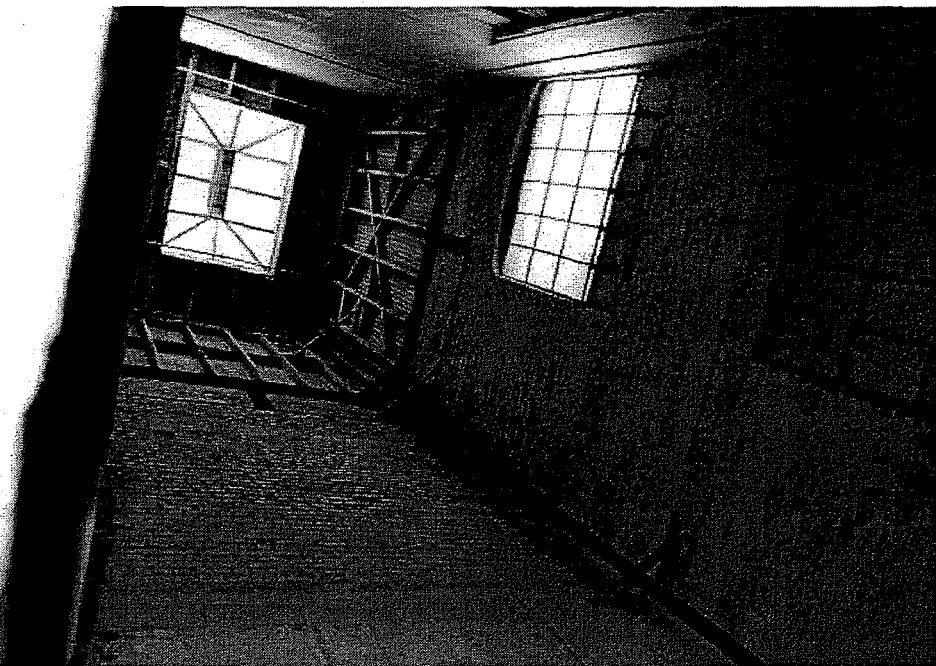
Figure 10: Interior shaft space at southeast corner of building. Second-story window at south façade picture right. Skylight at roof level pictured left. Facing south.
