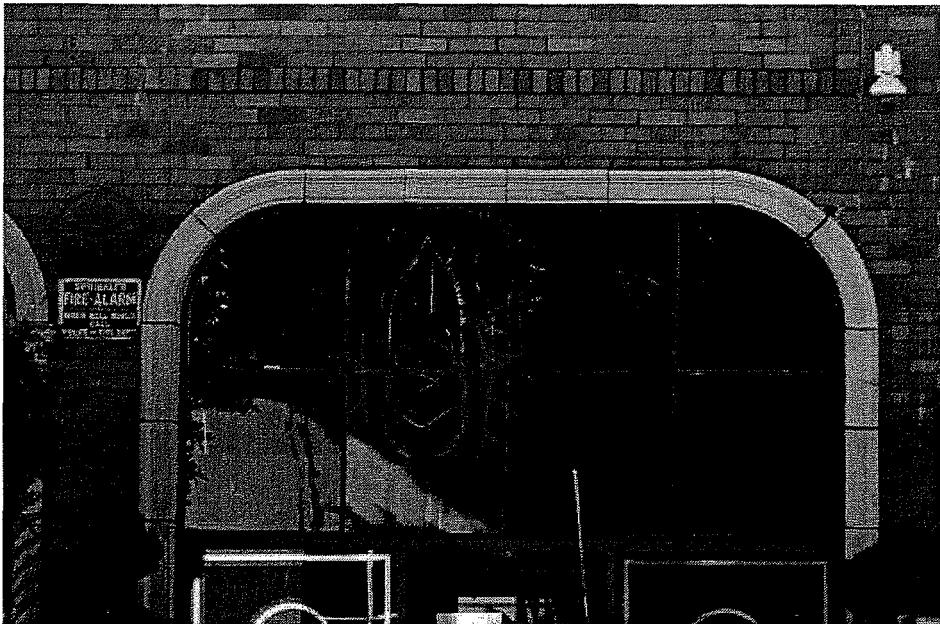
Figure 3: Divided-light transom above entry door in western bay, primary façade. Looking south.
