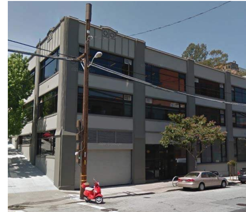
FRAME AND INFILL WITHIN DISTRICT 1005 Sansome St.
