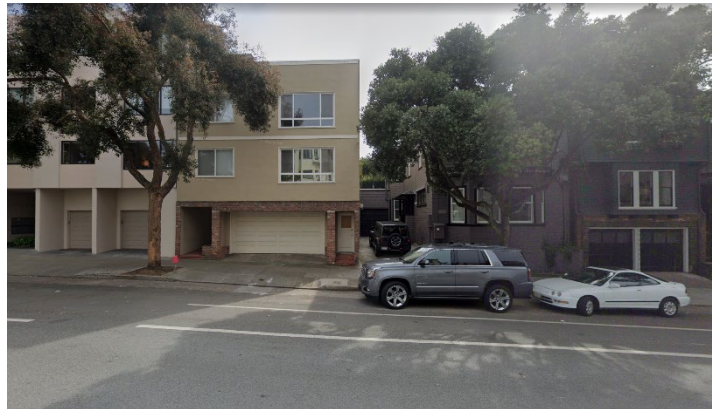
A 4-unit interior lot building adjacent to a 15-unit building (left) and a single-family home (right) in an RH-2 District in the Inner Richmond
