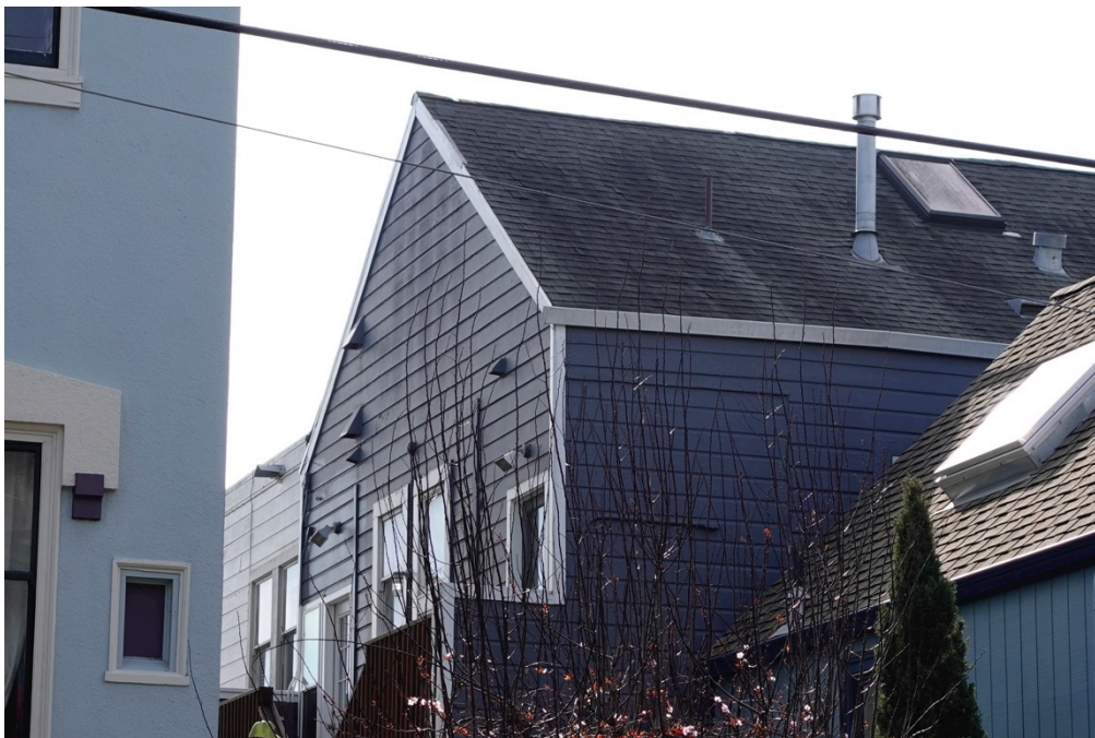
Figure 23: View of rear north elevation roof looking S (Garavaglia Architecture, 2023).
