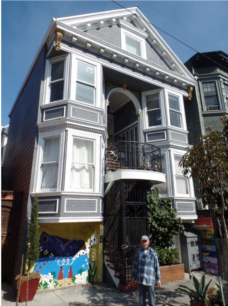
Figure 21: West elevation view of building looking SE. Ground level is considered a soft story (Garavaglia Architecture, 2022).
