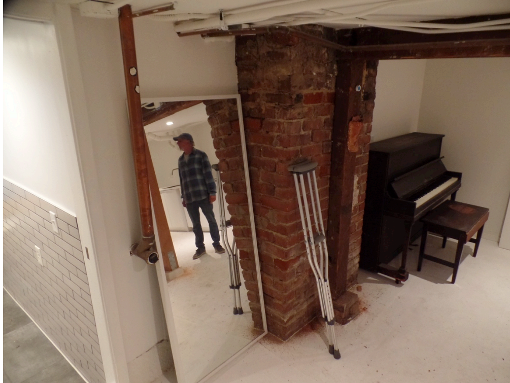
Figure 9: View of original brick chimney foundation (Garavaglia Architecture, 2022).
