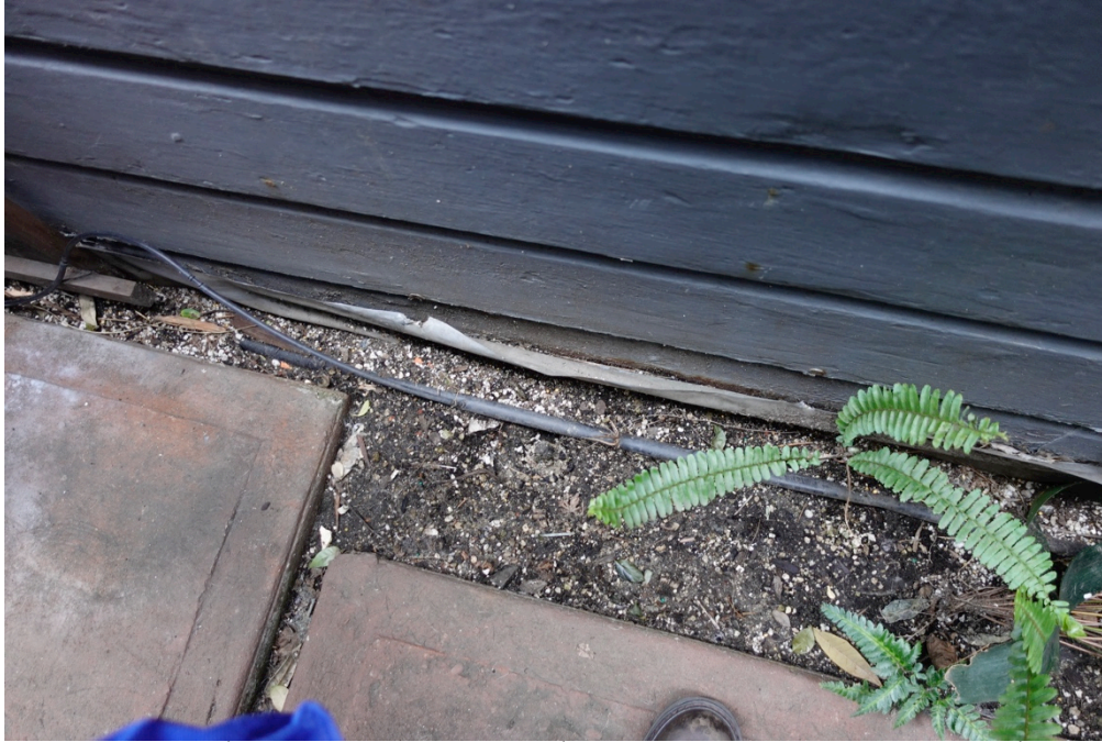
Figure 13: North elevation view of earth-wood contact (Garavaglia Architecture, 2023).
