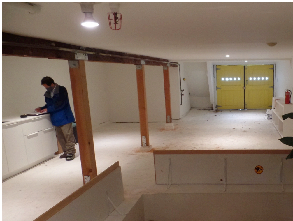
Figure 10: View of previous partial pier and post foundation work (Garavaglia Architecture, 2022).
