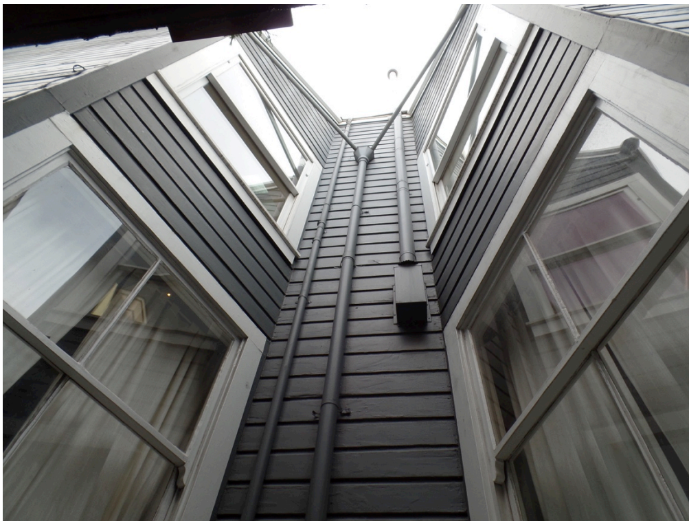
Figure 8: North elevation view of window alcove (Garavaglia Architecture, 2023).
