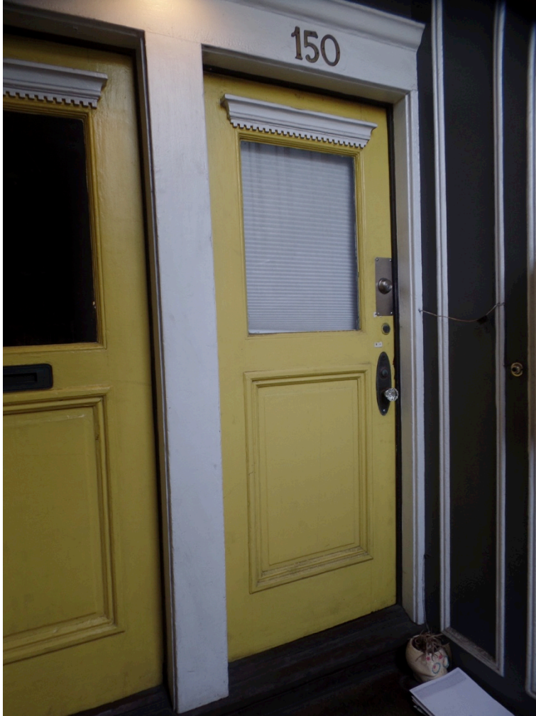
Figure 24: Exterior view of front door to Unit 150 (Garavaglia Architecture, 2023).
