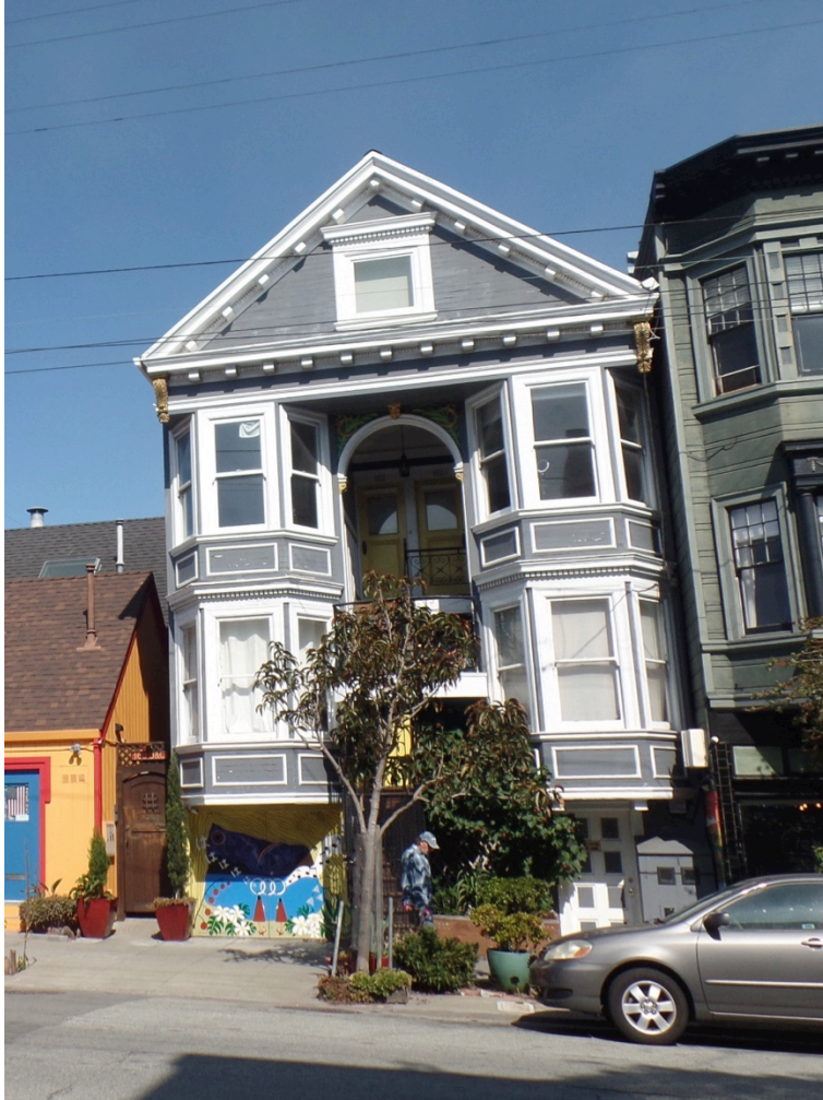
Figure 20: West elevation view of building from across Fillmore Street. Ground level is considered a soft story (Garavaglia Architecture, 2022).
