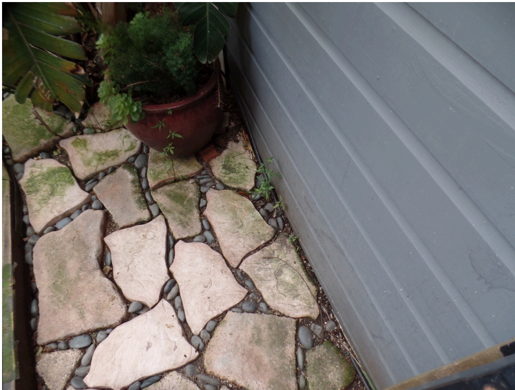
Figure 14: North elevation view of earth-wood contact (Garavaglia Architecture, 2023).
