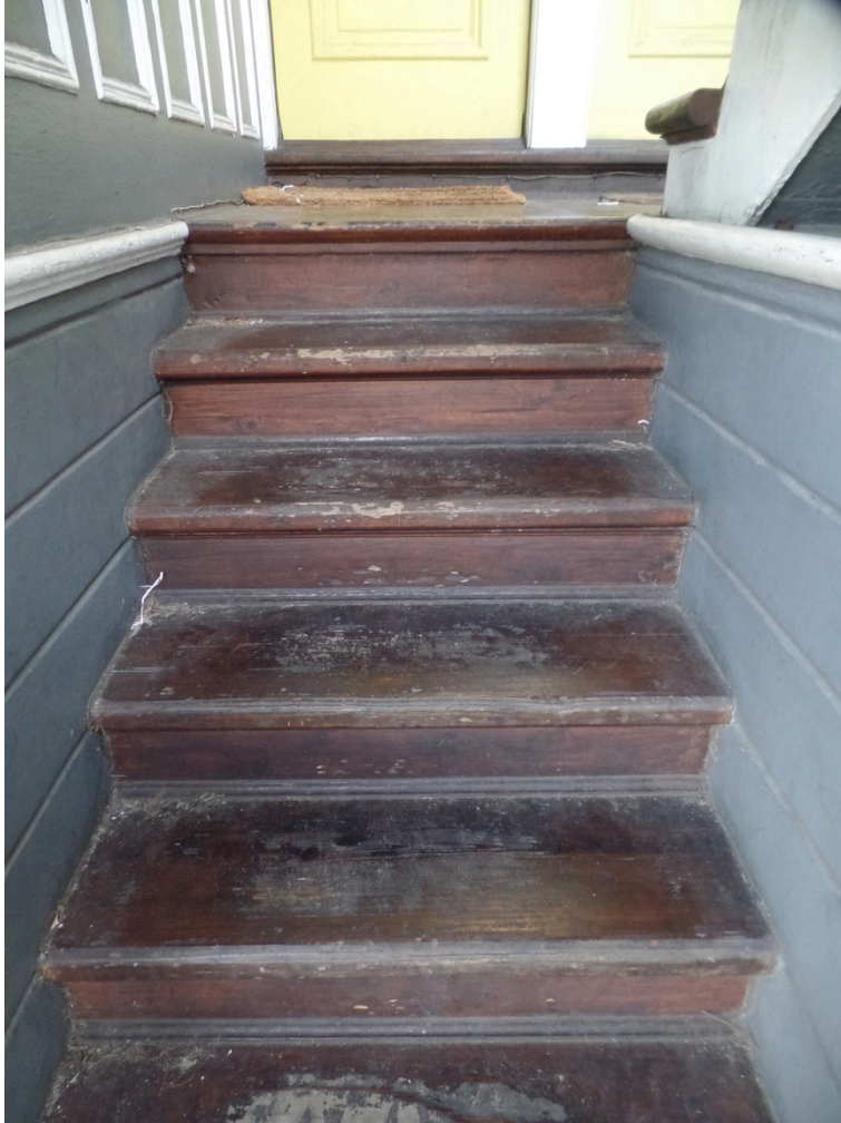
Figure 16: View of front entry stairs to second level (Garavaglia Architecture, 2023).
