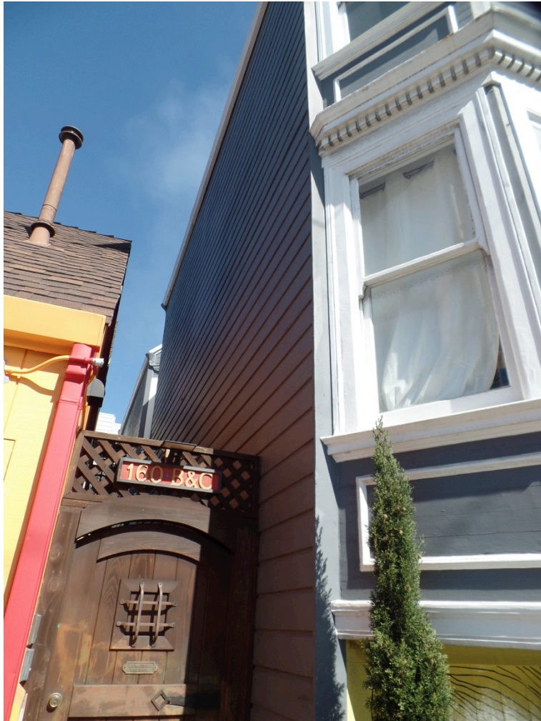
Figure 6: North elevation view from sidewalk on Fillmore Street (Garavaglia Architecture, 2022).
