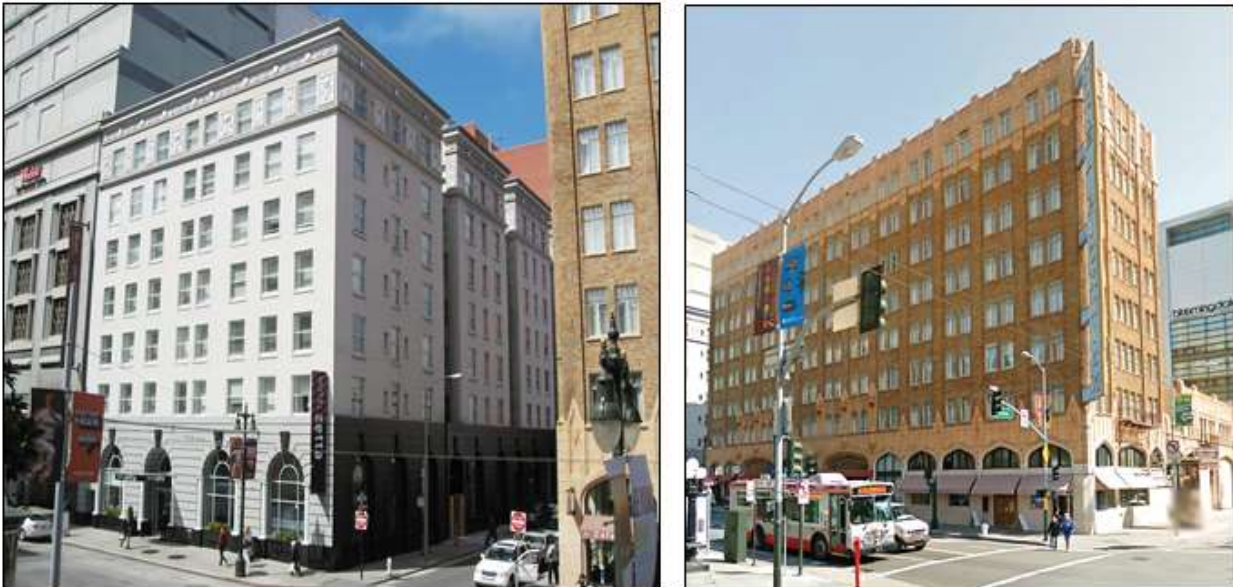
The Hotel Lankershim at left, and the Pickwick Hotel at right (Google Maps)
