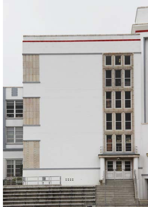
Figure 22. East part of south façade; view toward north.
