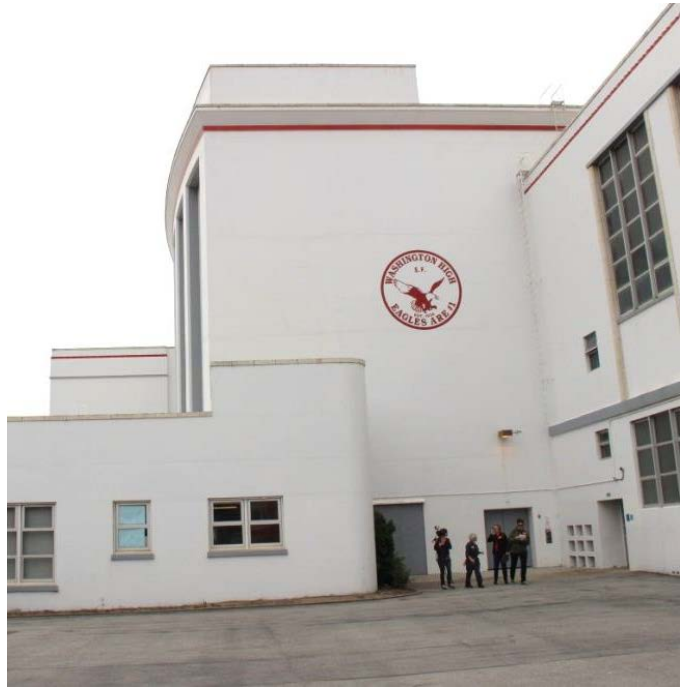
Figure 45. East façade of the Auditorium; view toward west. The music room addition is visible to the left and the gymnasium to the right.
