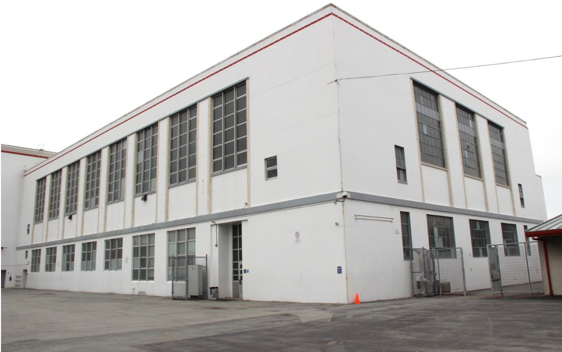
Figure 41. Gymnasium, south and east façades; view toward northwest.
