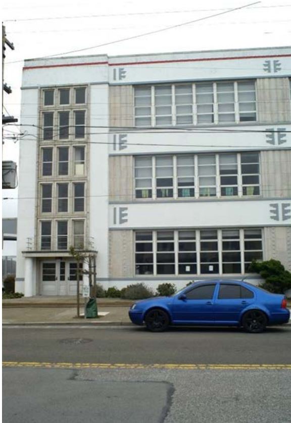
Figure 12. Primary façade, first and second bay; view toward east.
