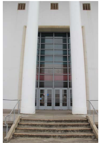
Figure 44. Main entrance to the Auditorium.
