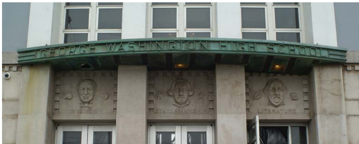
Figure 16. Canopy and bas-relief panels above main entrance.
