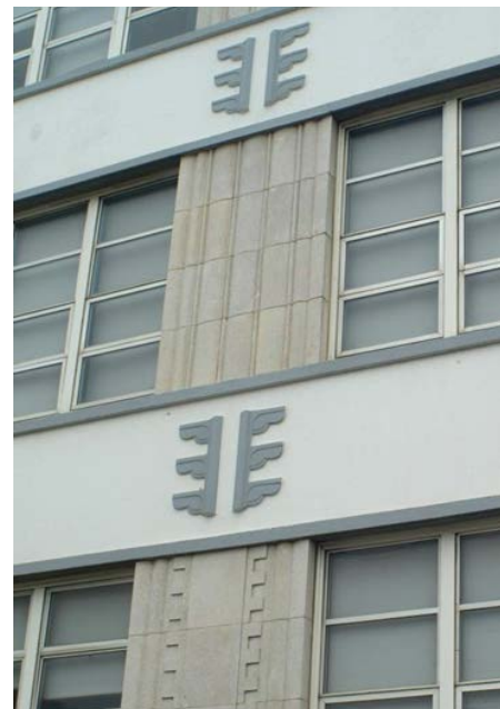
Figure 14. Primary façade, detail of piers, molding, and "tree and leaf" bas-relief ornament; view toward east.
