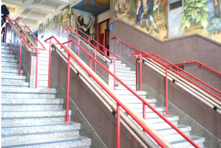
Figure 29. Stairs accessing main lobby; view toward southwest.
