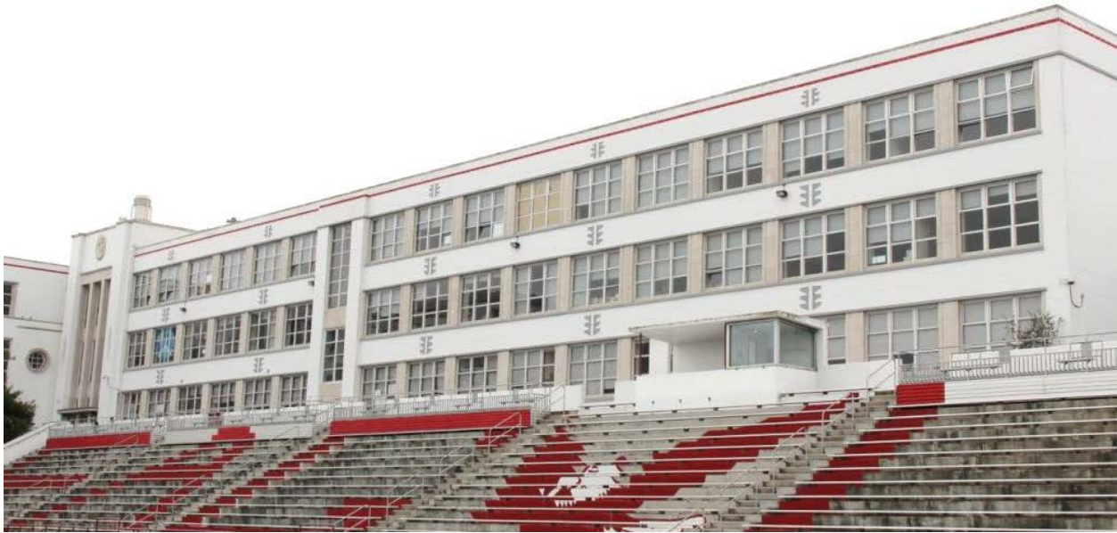
Figure 26. East façade of the academic building; view toward southwest from football field.
