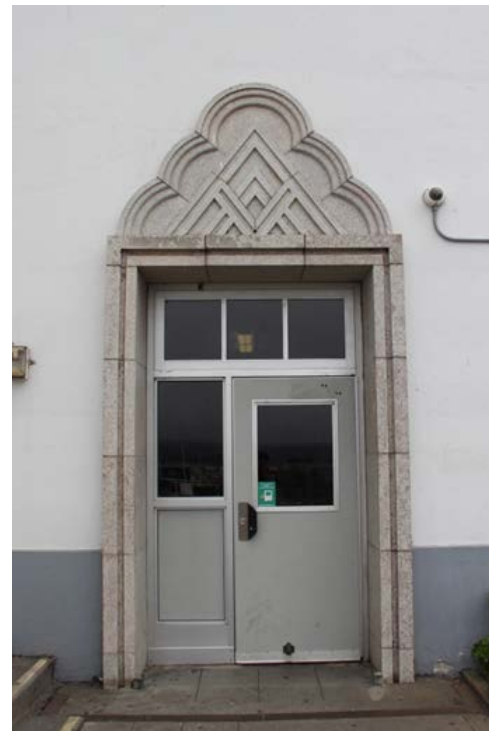
Figure 23. Main entrance on north façade.
