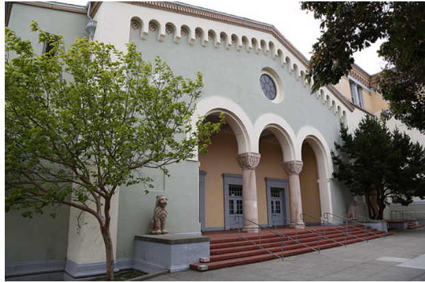
Figure 7. Presidio Middle School auditorium; view toward southeast.
