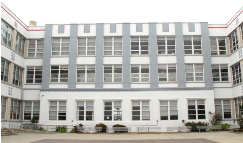
Figure 20. Central part of south façade; view toward north.
