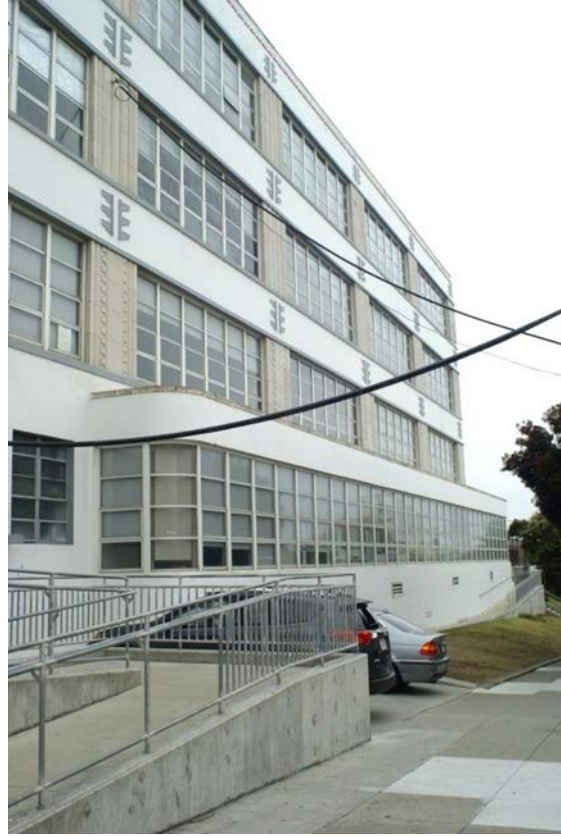
Figure 18. Primary façade, 12 th through 16 th bays; view toward southeast.
