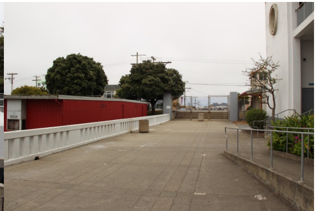
Figure 59. Detail of the esplanade, north of the gymnasium, with modular classrooms at left; view toward east.
