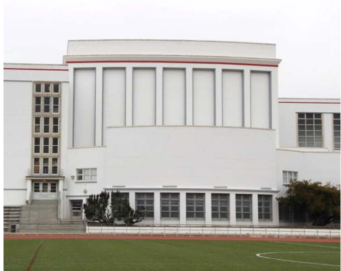
Figure 46. South façade of the Auditorium; view toward north. The academic building is visible to the left and the gymnasium to the right.
