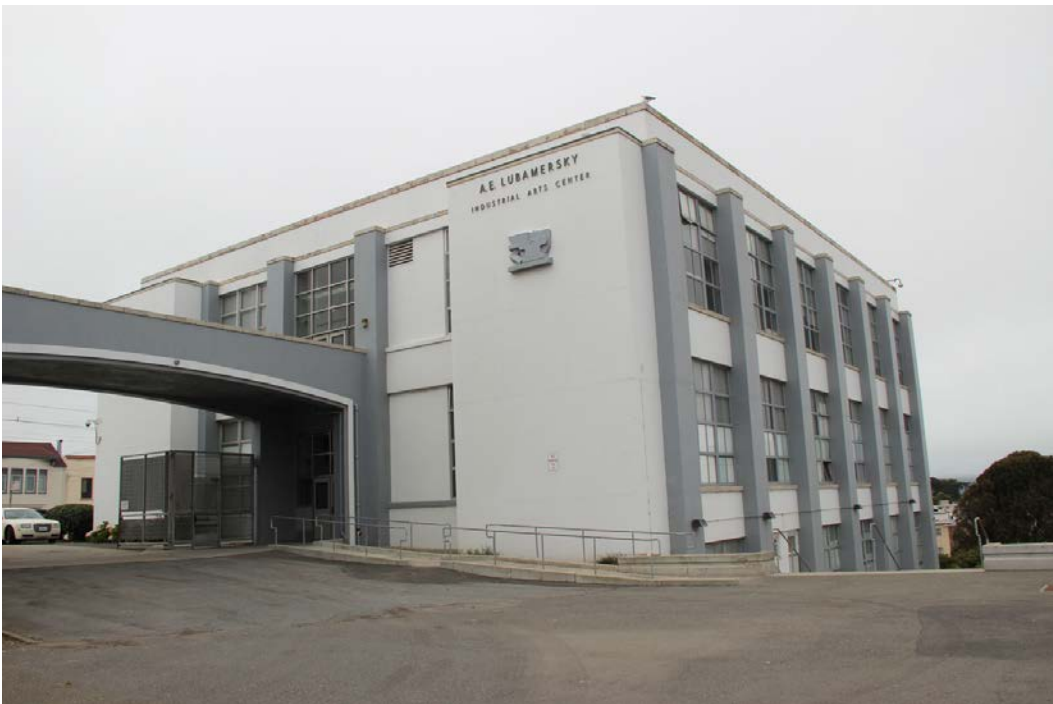
Figure 37. South façade of shop building; view toward northwest.
