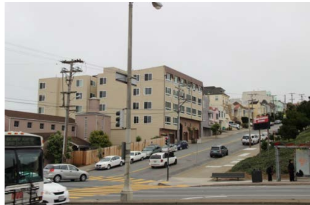
Figure 5. Contractor Modern apartment building at 524 30 th Avenue, constructed 1971; view toward southeast.
