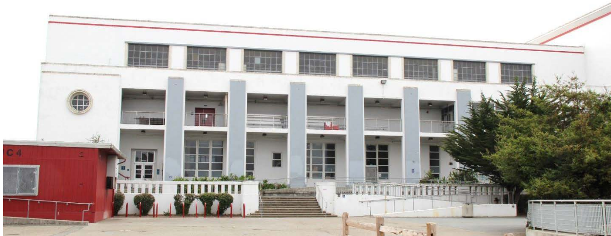
Figure 40. Gymnasium, north façade; view toward south.
