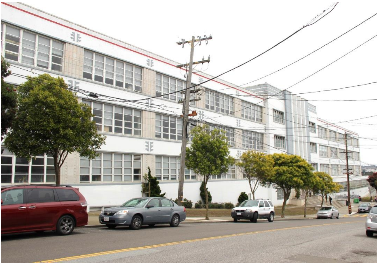
Figure 11. Primary façade of academic building; view toward southeast.
