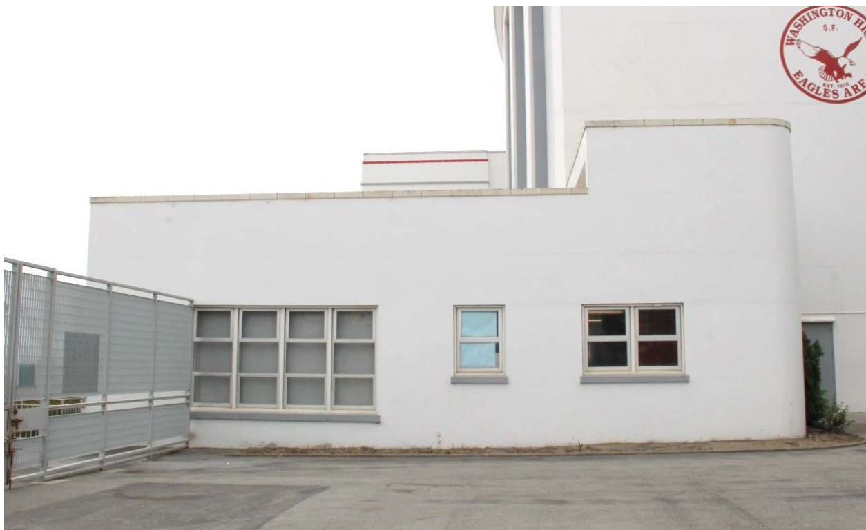
Figure 51. East façade of the music room addition; view toward west.
