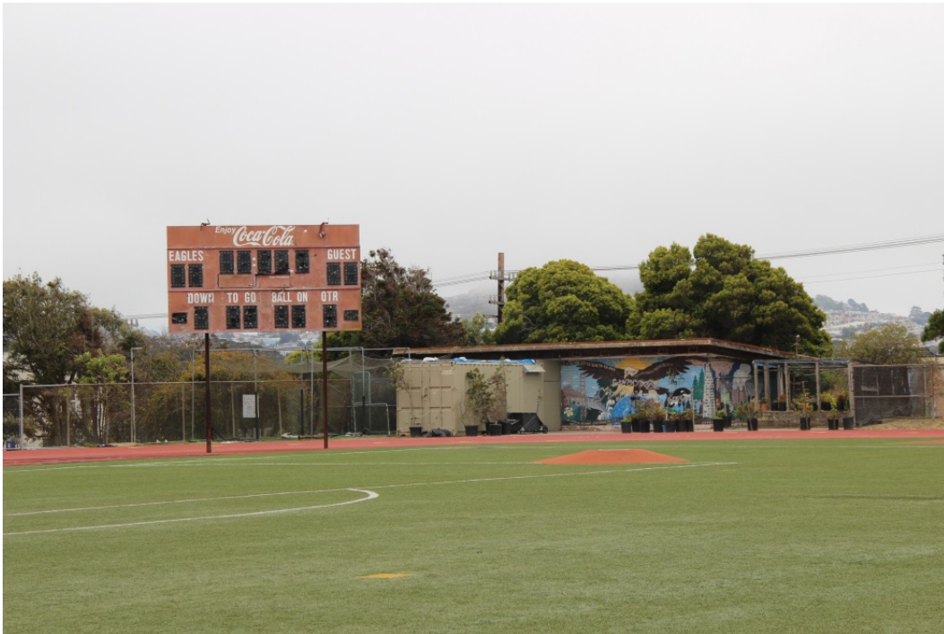
Figure 62. Equipment shed southeast of the track; view toward south.
