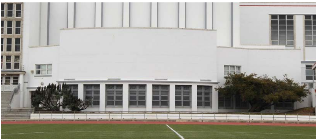
Figure 50. South façade of the music room addition; view toward north.
