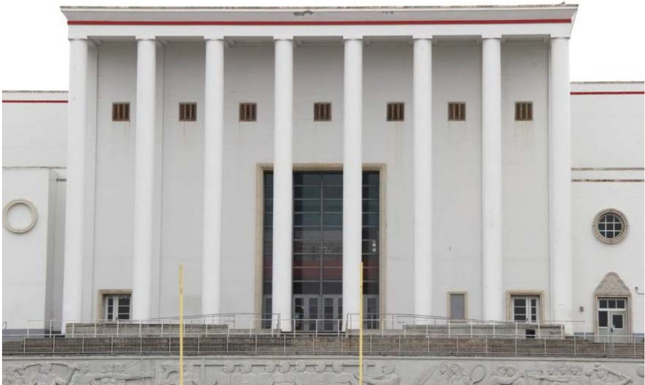
Figure 43. North façade of the Auditorium; view toward south.
