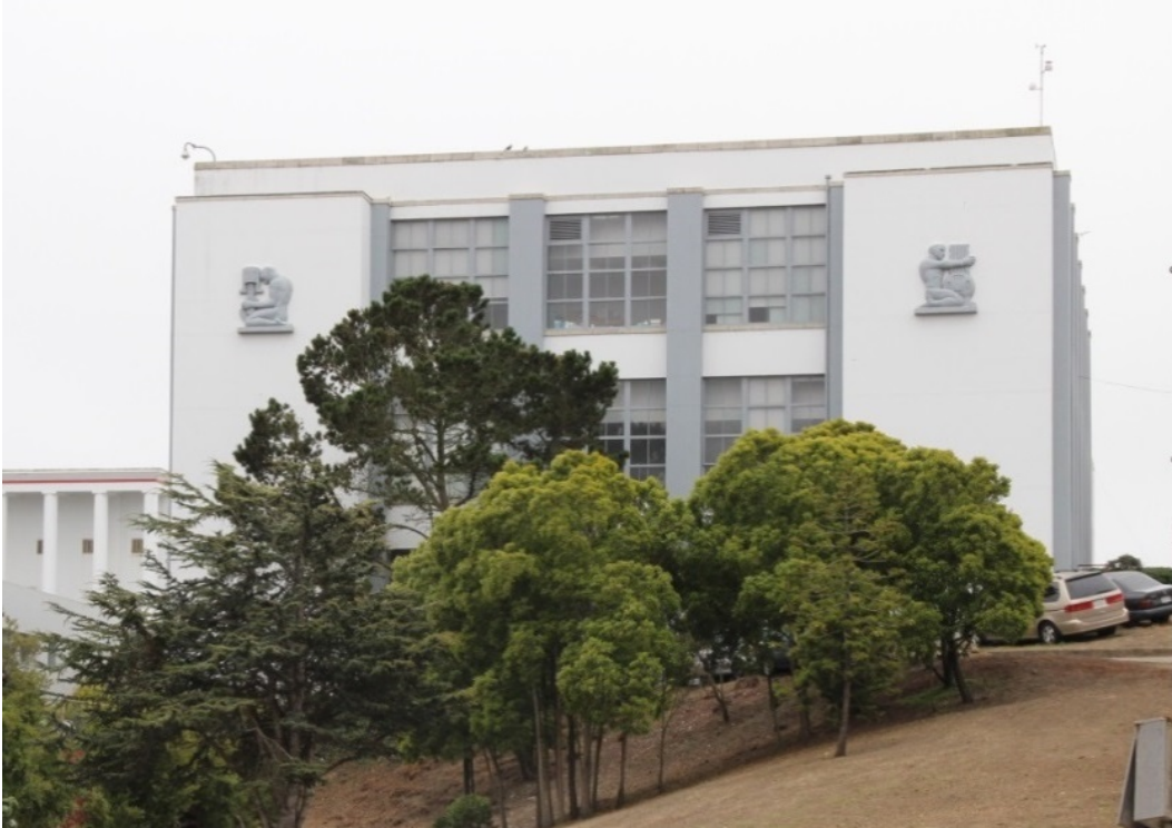
Figure 36. North façade of shop building; view toward south.
