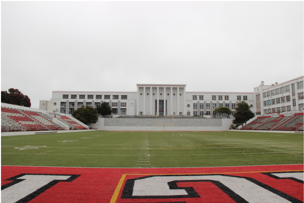
Figure 54. Football field and bleachers; view toward south.
