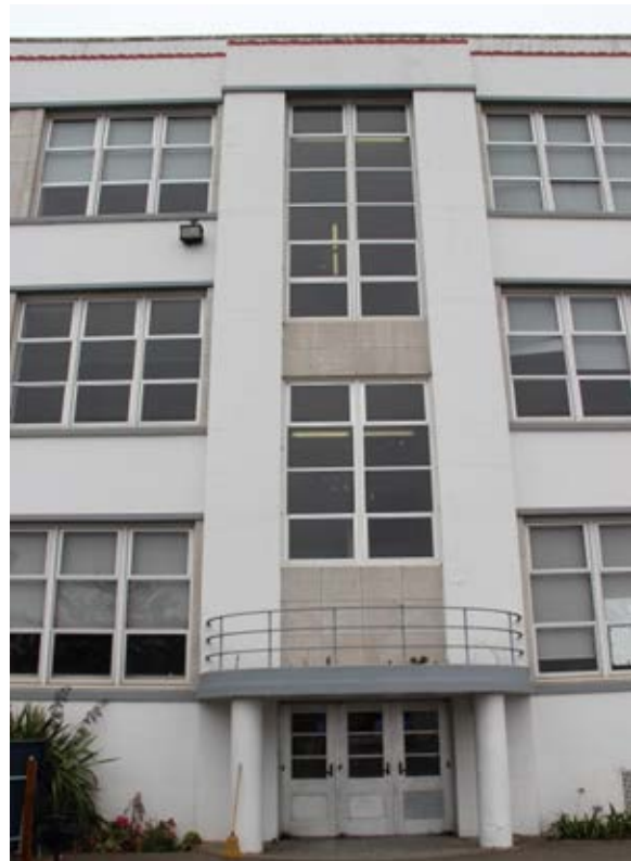
Figure 28. Entrance pavilion in eighth bay of east façade; view toward west.
