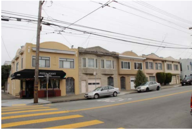
Figure 2. Mediterranean-style rowhouses at the northeast corner of 32 nd Avenue and Balboa Street, constructed 1920; view toward northeast.
