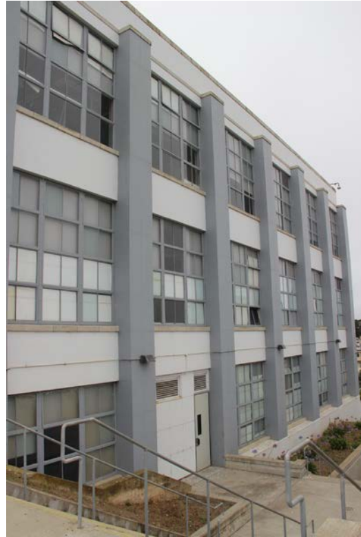
Figure 35. East façade of shop building; view toward north.
