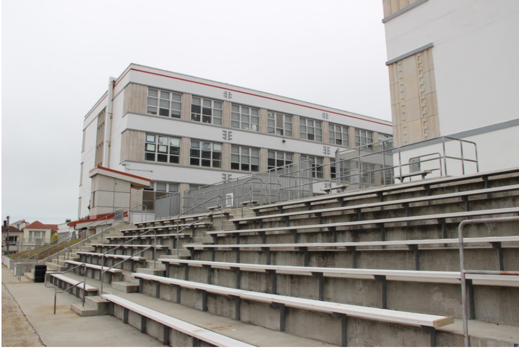
Figure 61. Bleachers and wheelchair lift tower; view toward west.
