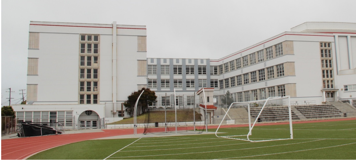
Figure 19. South façade of the academic building; view toward northeast.
