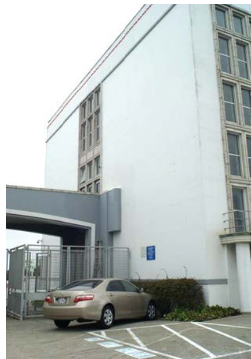
Figure 25. North façade, west section; view toward southeast.
