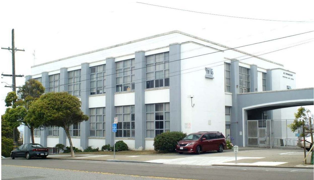
Figure 34. West façade of Shop Building; view toward northeast.
