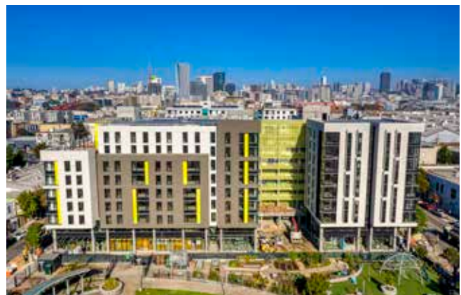
Casa Adelante (2060 Folsom): all-electric affordable housing with 127 affordable apartments, and 29 units for formerly homeless transitional-age youth. Developed by MEDA and Chinatown CDC. Photo credit: James E. Roberts-Obayashi Corp. (general contractor)
