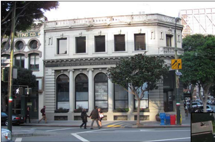
View facing east at 700 Montgomery Street
