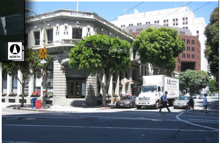
View facing east at 700 Montgomery Street
