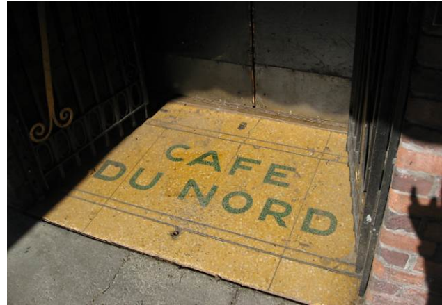
Detail of terrazzo threshold
