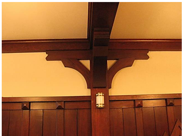
Detail of trim work in the first floor meeting room.
