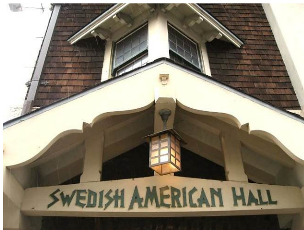
Gable hood above the main entrance to the hall
