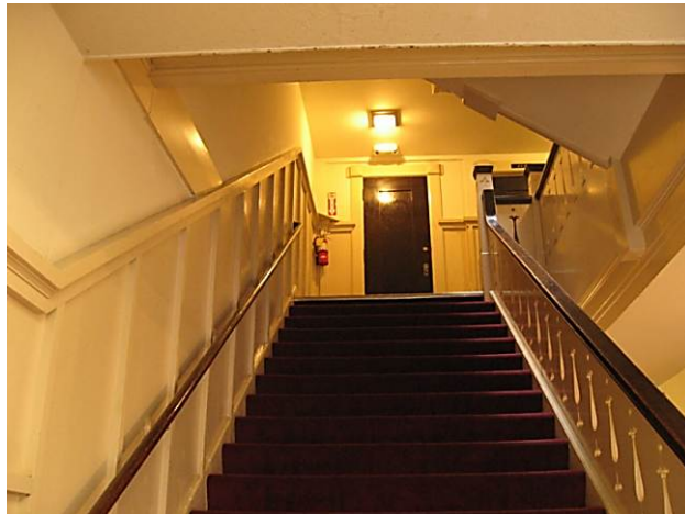
View north up the stairs from the main entry to the second floor landing.
