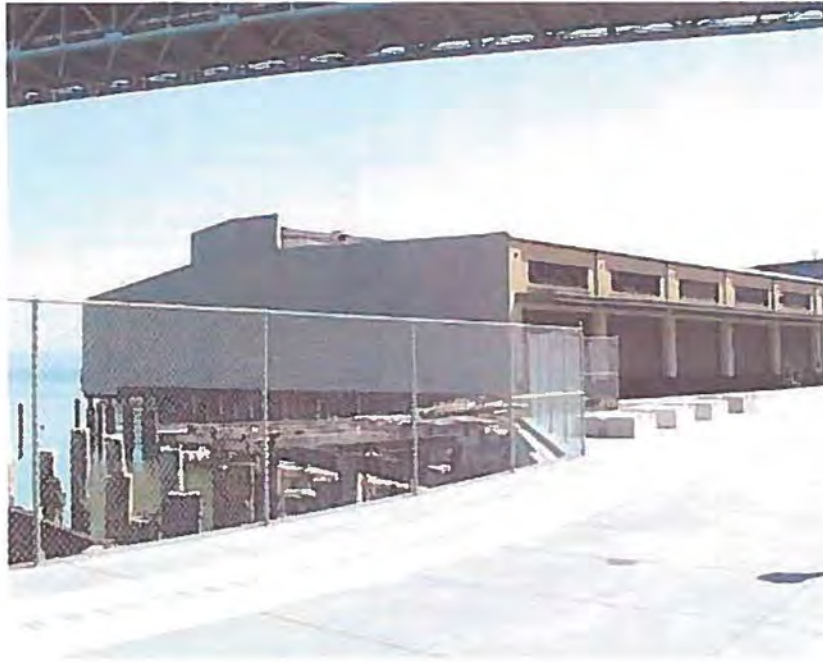
Photo 1: North end wall and partial west elevation of Pier 24 Annex
