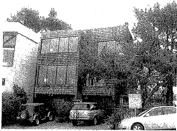
Figure 4. North façade Source: KVP Consulting
