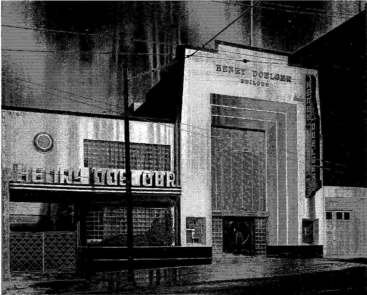
In 1940, the original building was expanded to include a horizontal addition at west facade. Source: History Guild of Daly City/Colma (Portola Studio, circa 1940).
