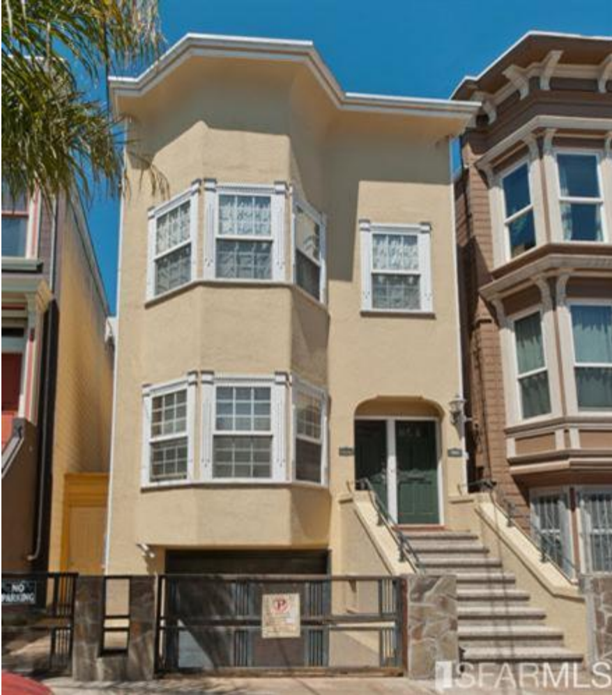
Figure 1. Before image of 354-356 San Carlos St. taken in 2012. Front facade view looking east.
