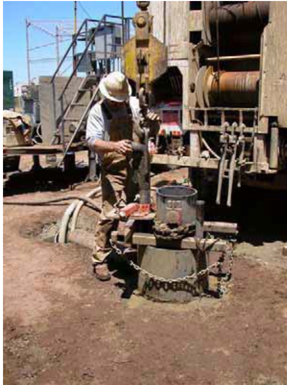
Figure 2.7 San Francisco Groundwater Supply Test Well Drilling
