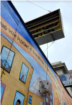
new attempted splicing today of electric wires at church mural
