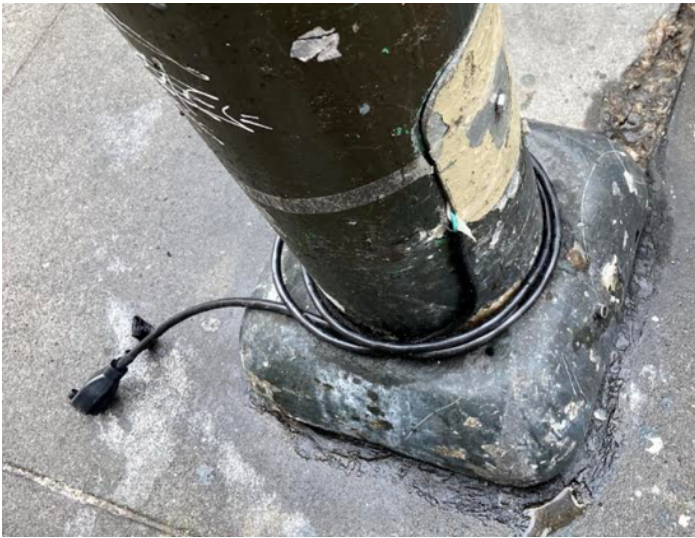
new lamppost splicing - after PG&E repair
