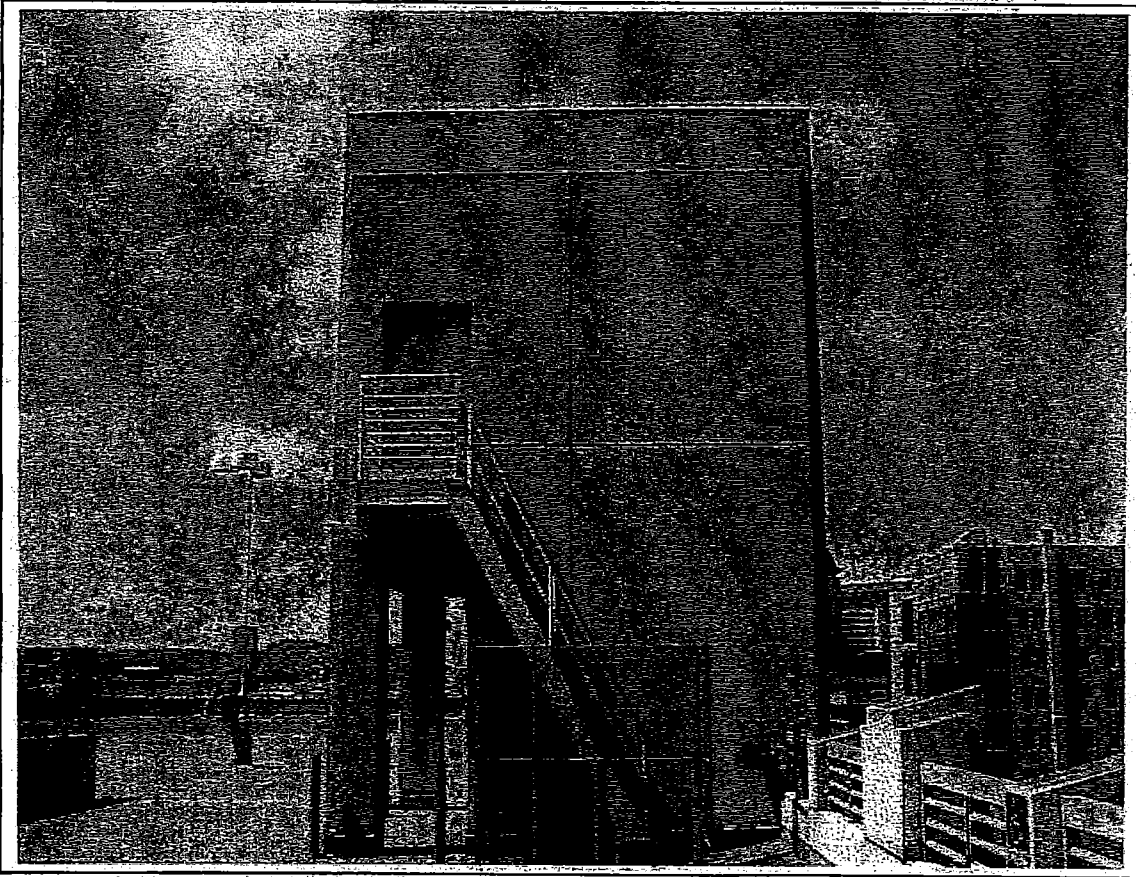
Photo of elevator/stairway structure. Proposed antenna to be placed on top via sled/ballast mount.
