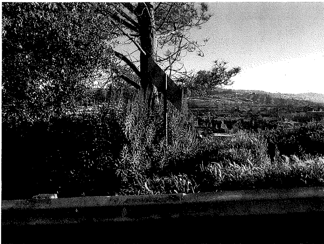
30-foot pine tree growing above PG&E Gas Transmission Pipeline 109 at Bernal Heights Blvd. - in violation of PG&E's threatening the pipelines protective coating.
