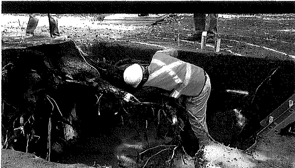
Example of incompatible vegetation planted within the ROW.
