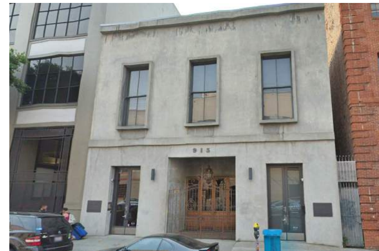
PROJECTED WINDOW FRAME WITHIN DISTRICT 915 Battery St.
