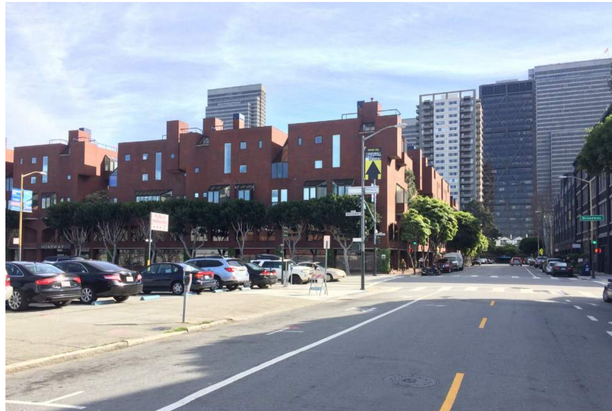
VIEW 1 LOOKING SOUTH ON FRONT STREET
